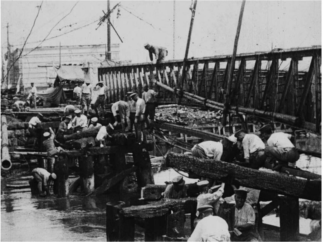
Fig.5 Restoration work on Umibe Bridge.
