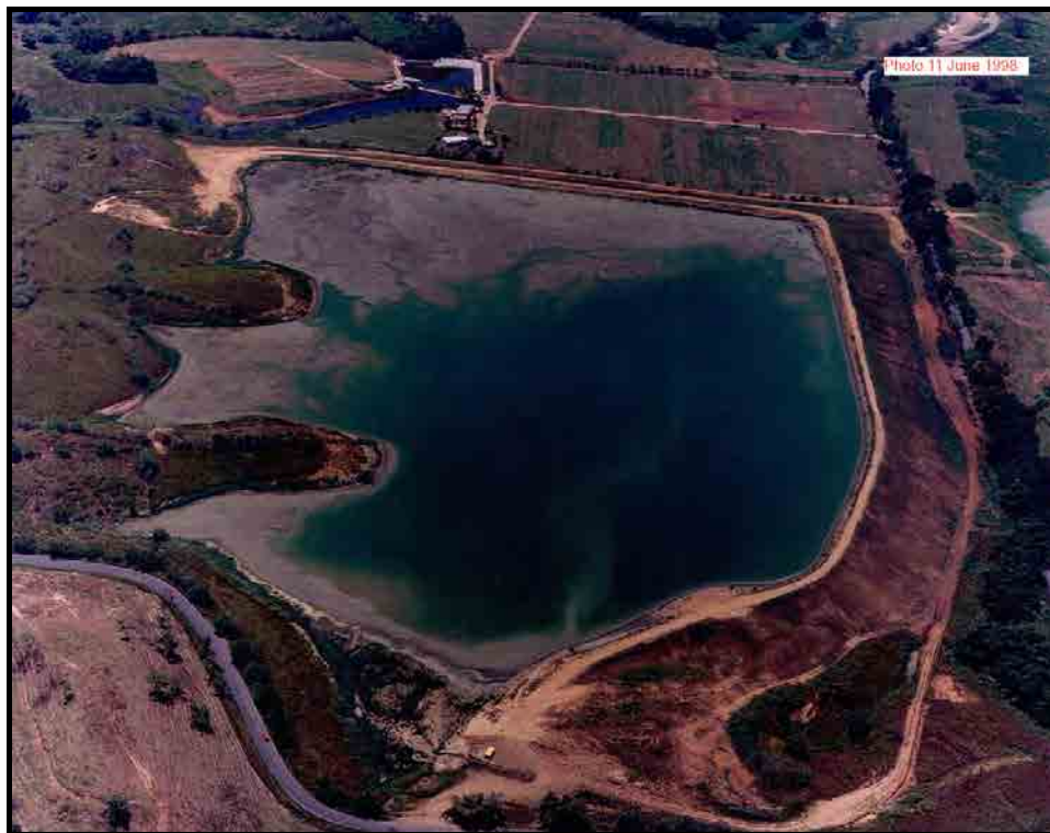
Figure 2. Historic picture of Dike B.
