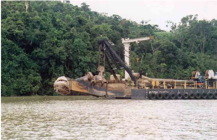
Hydraulic Dredging Barge
