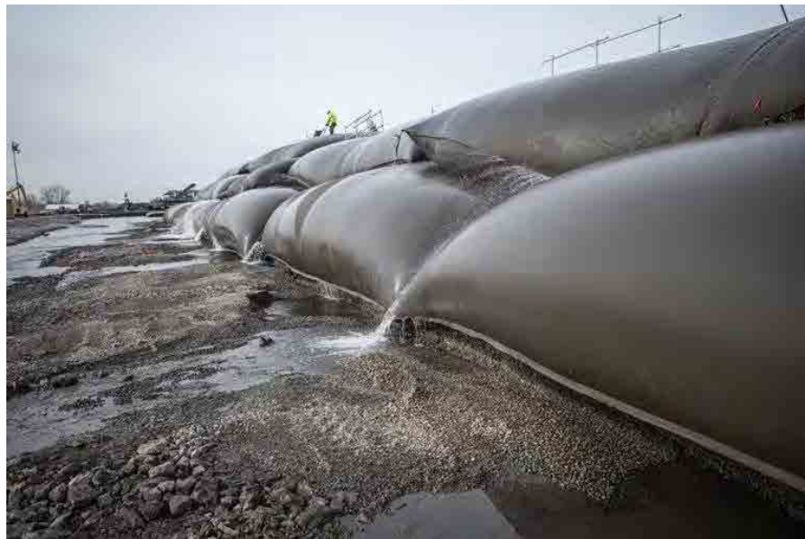
Geotextile Tubes Dewatering System
