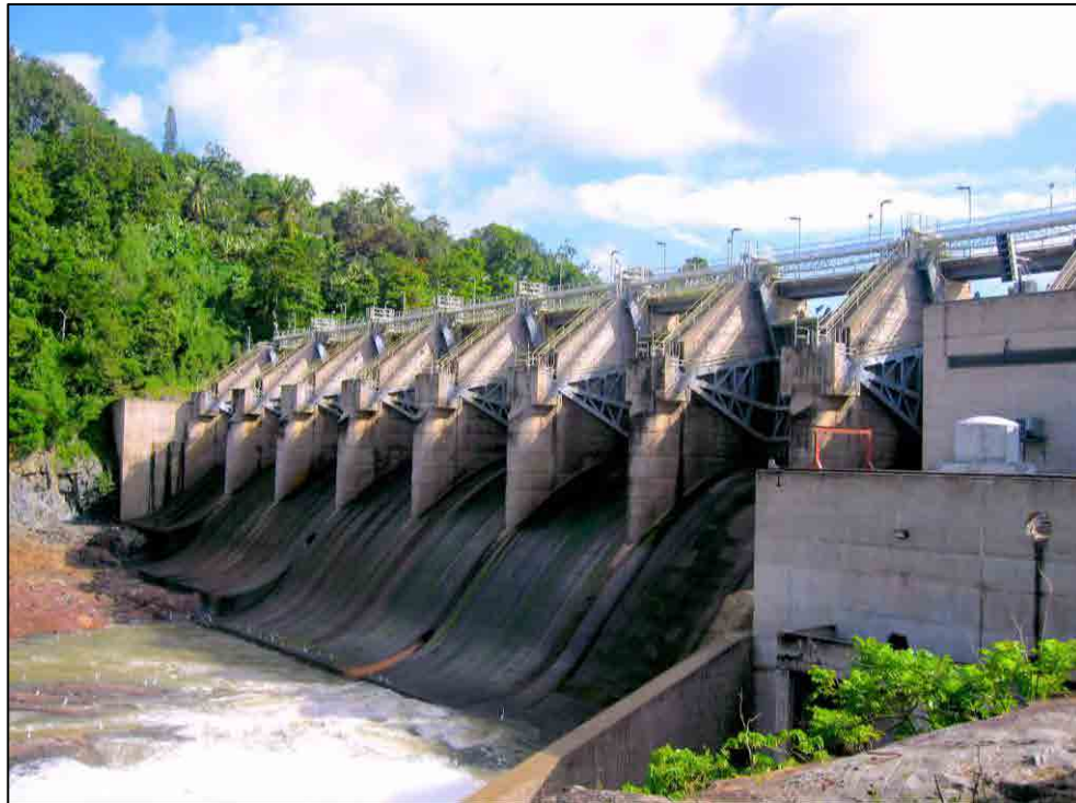
Figure 3: Photograph of downstream face of Loíza dam.
