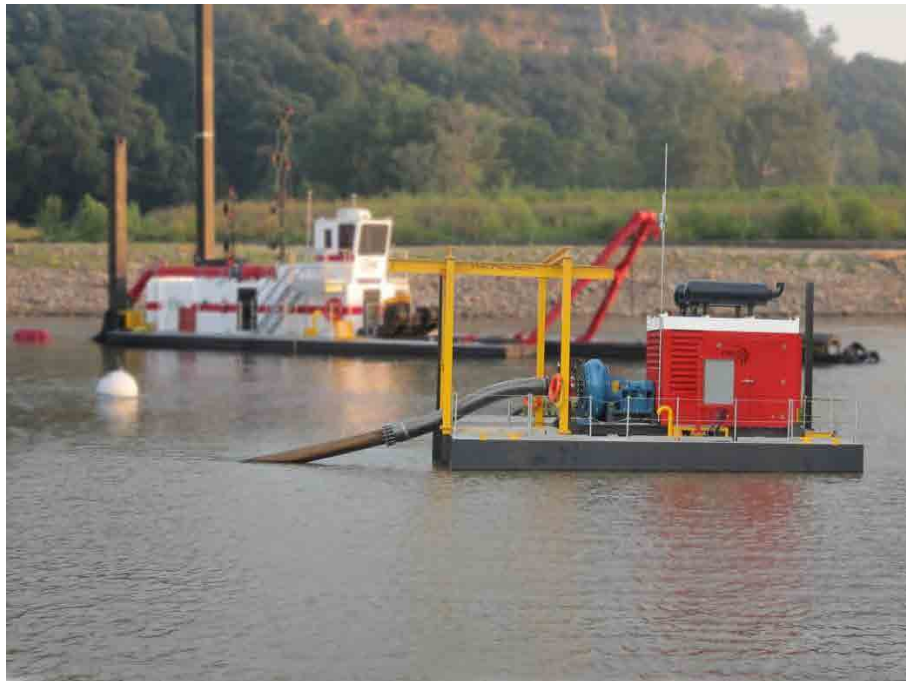
Floating Booster Pump Station
