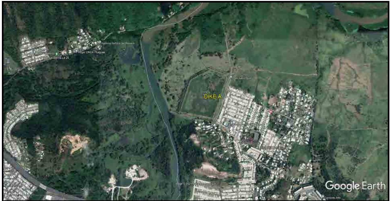
Figure 1. Location of Dike A.
