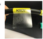
Step 3: Apply pressure to end of "tail" to ensure adhesive bond -Job done!
