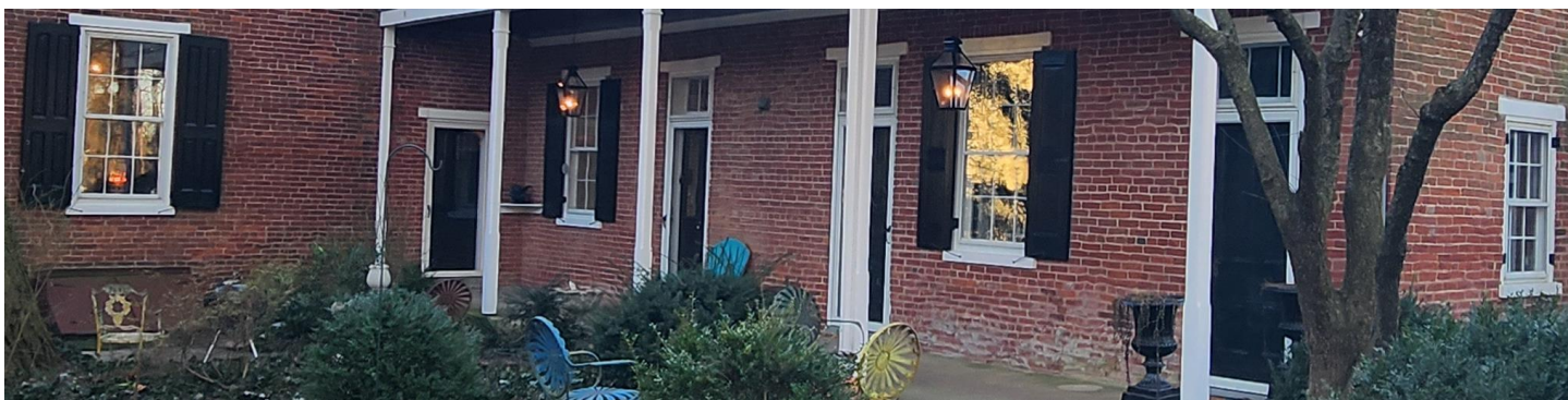
The first story in the back of the house six by six windows with panel shutters.
