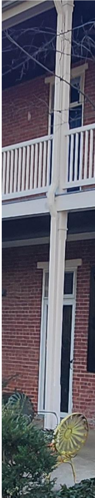
The house has columns at the back of the house that support the second story porch.
