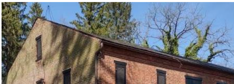
The roof of the guest house is a gable roof made of slate.
