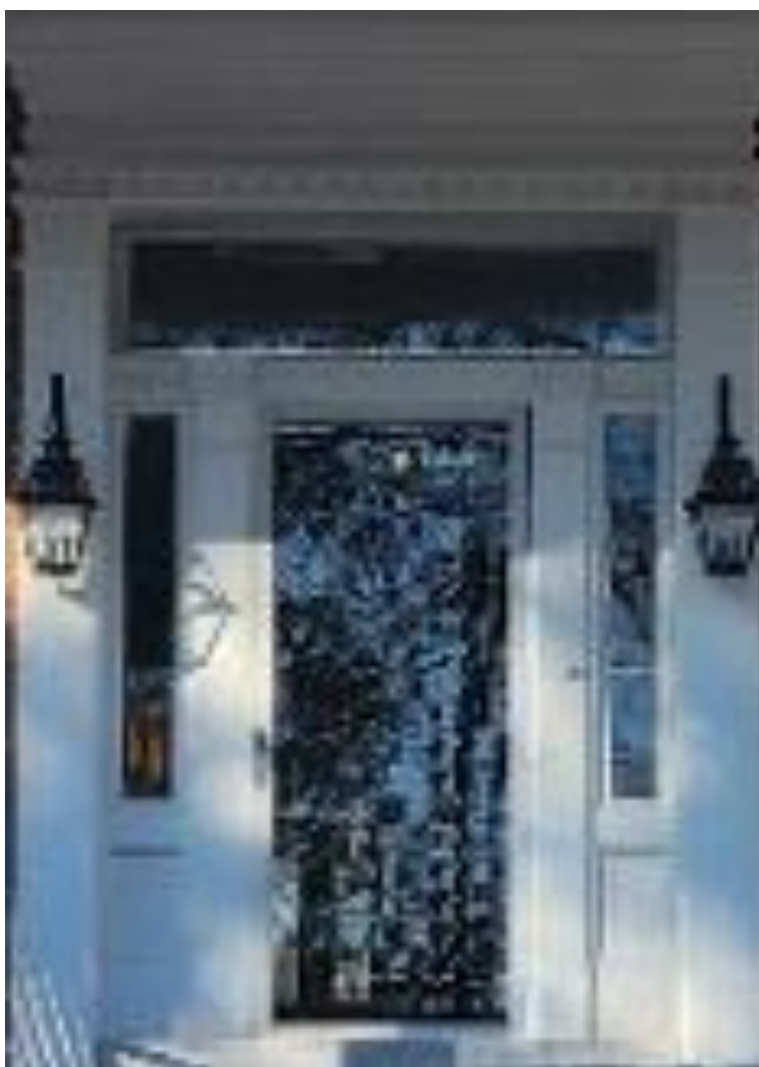
The house has a transom with two sidelights with one at each side.
