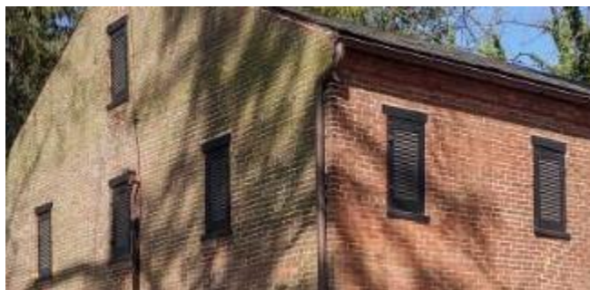
The guest house has louvered shutters on the front and side walls on the second story.
