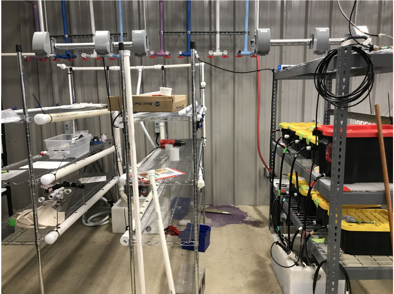
Figure 4. New invertebrate racks at SMARC under construction.
