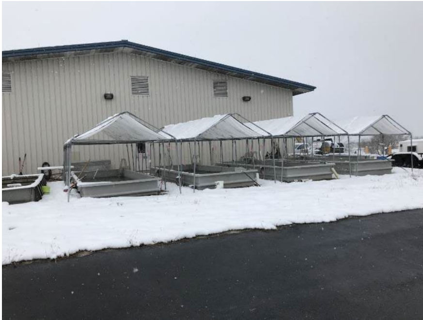
Figure 20. Shade structures installed over the Texas wild rice tanks at the Uvalde National Fish Hatchery.
