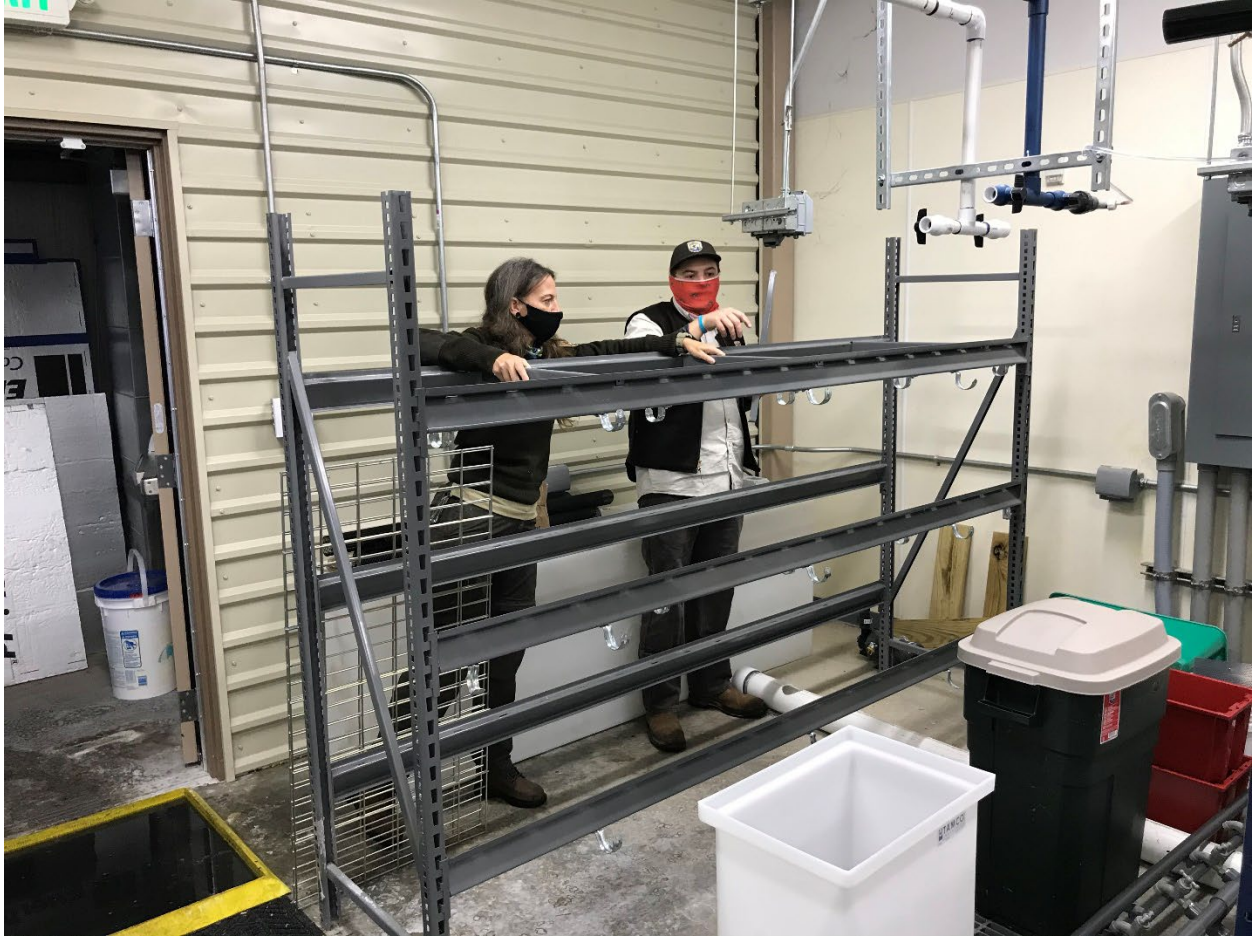
Figure 2. Jennifer Whitt and Benjamin Thomas assisting with the construction of the new hospital rack in the UNFH refuge room.
