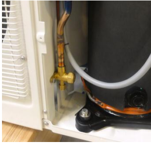
Figure 22: Liquid line service port
