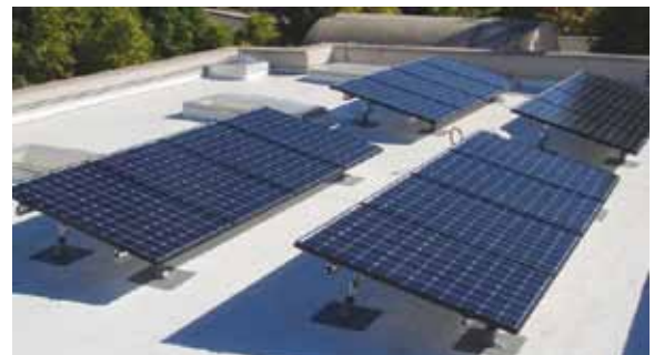
Installation with Tilt Hardware Kit
