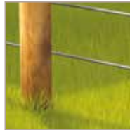
No vegetation - no contact between the vegetation and the fence wire
