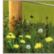
Heavy vegetation - the wire runs completely in vegetation
