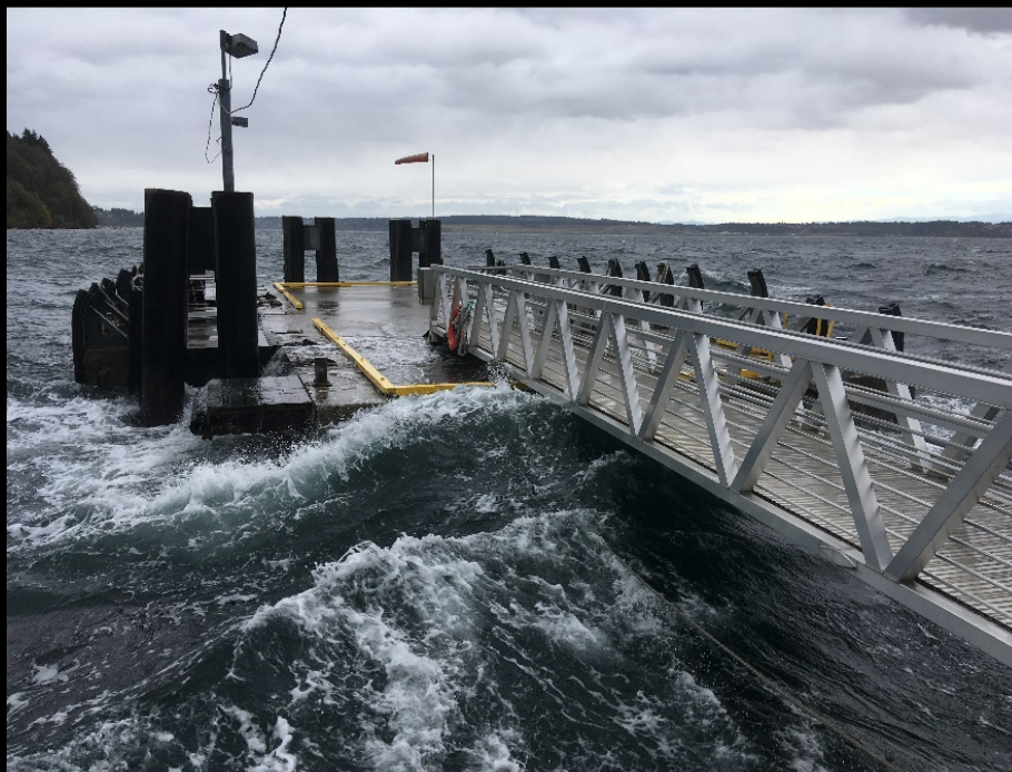
The ramp & dock can be hazardous in rough seas & inclement weather.
