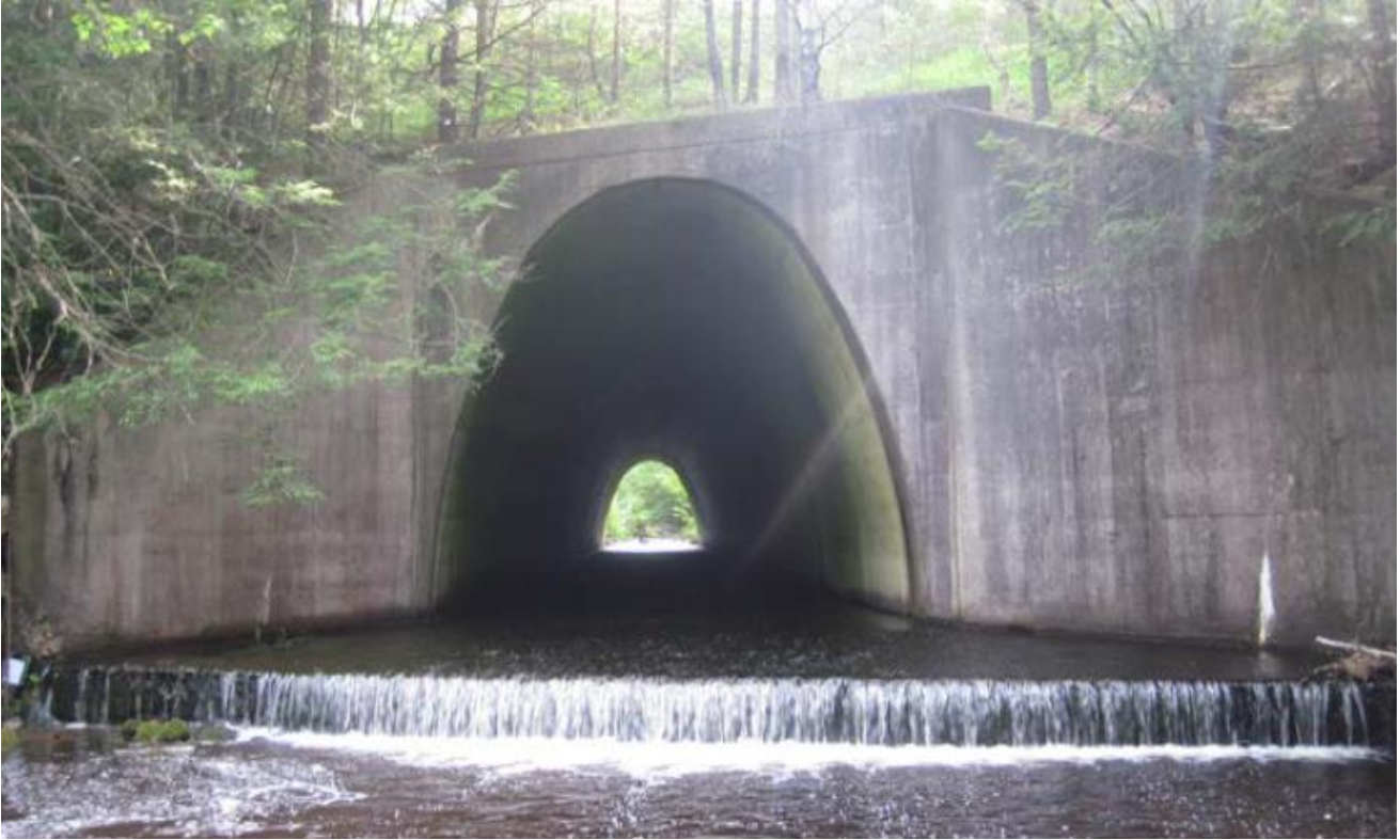
Structure Type 33: Tied-Arch Culvert
