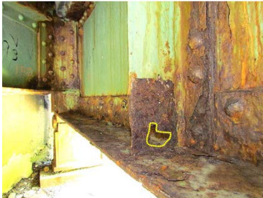
Figure 3.13 - Element 107: Girder, Steel CS-3.
