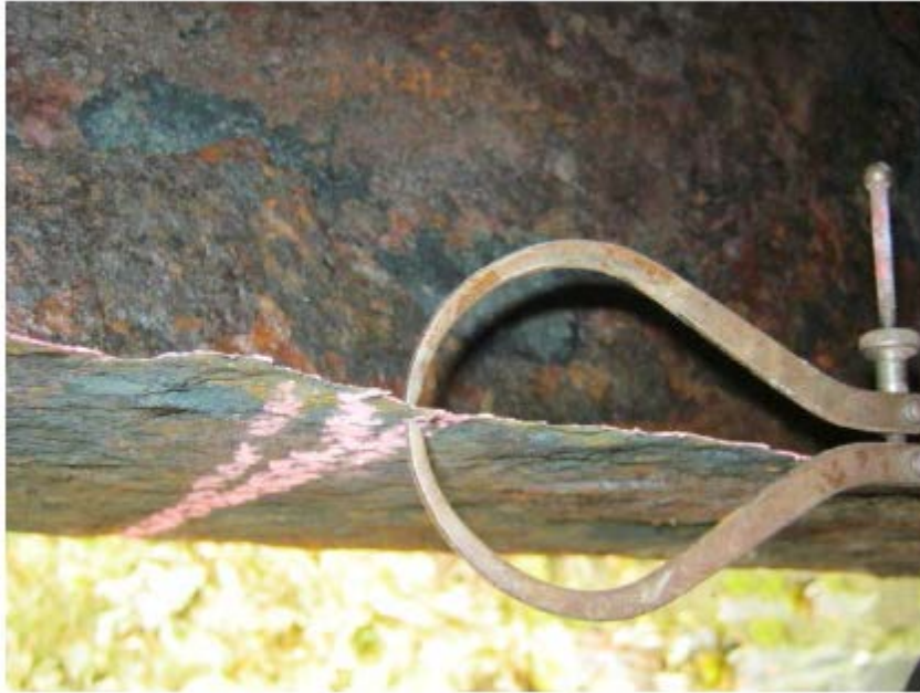
Figure 3.14- Element 107: Girder, Steel CS-4
