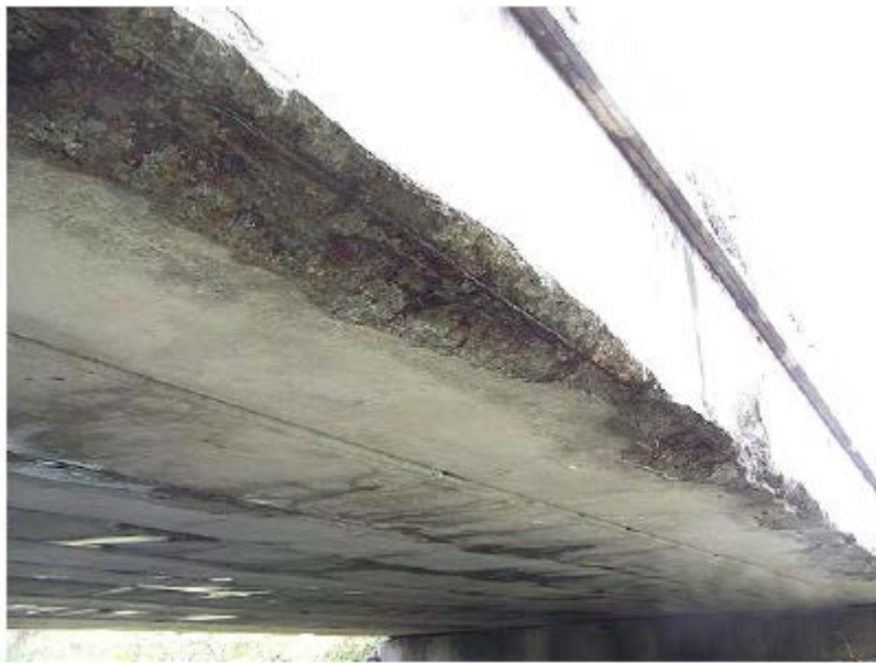
Figure 3.15 - Element 104: Box Girder, Prestressed Concrete CS-3
