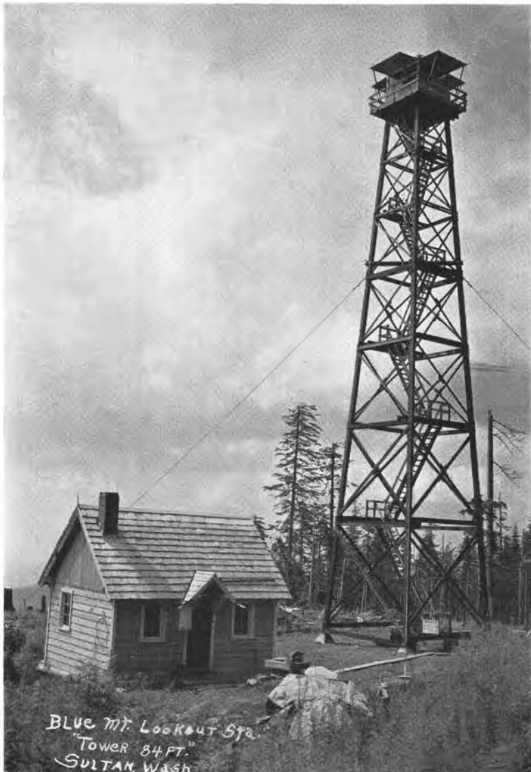
Blue Mountain Lookout Tower and Ground House, Snohomish County.
