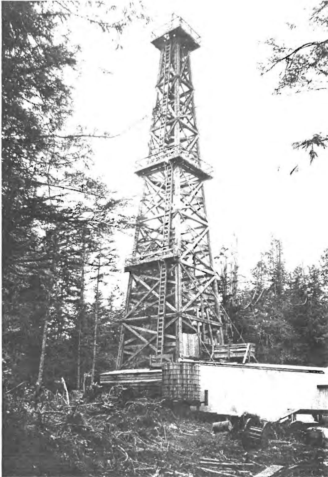
Wooden derrick of the Sims No. 1 well, circa 1931, drilled near the Jefferson oil seep in Jefferson County. Numerous exploratory wells have been drilled in this area and elsewhere on the western Olympic Peninsula and adjacent continental shelf. Photograph courtesy of Jones Photo Company, Aberdeen, Washington.
