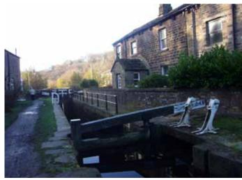
Inclined paddle gear on the Diggle Flight and beams on the non-towpath side © Howard Lunn
