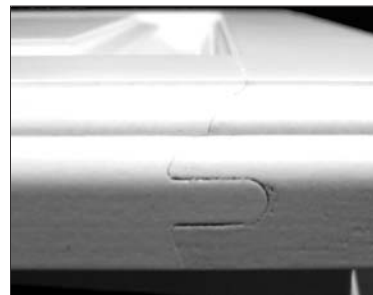
Example of end joint separation
