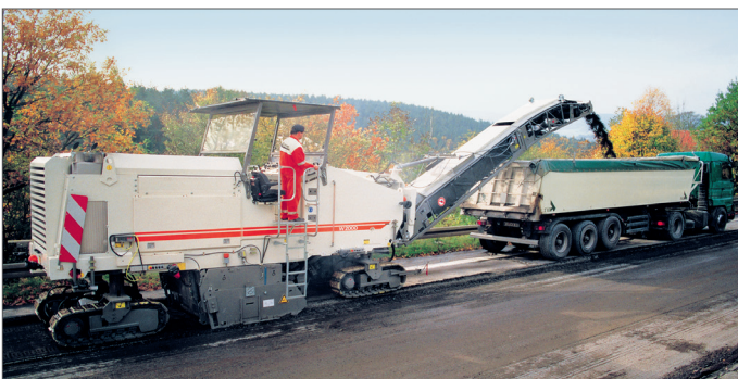
Road Milling Machine
