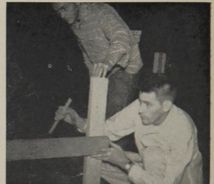
DAVE ARNETT and CHUCK STRAWMAN constructing foundation for Beta's Homecoming display.
