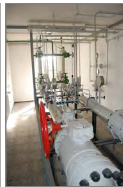
GAS PRESSURE REGULATION STATION WITH HYDROGEN INJECTION (E.ON TECHNOLOGIES)
