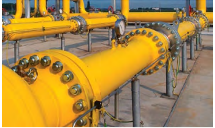
HYDEPLOY SAMPLE GAS NETWORK FOR THE TESTING OF NATURAL GAS/HYDROGEN BLENDS (SOURCE: ITM POWER)
