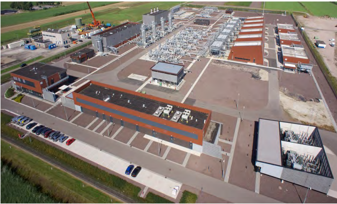
SURFACE FACILITY OF AN UGS
