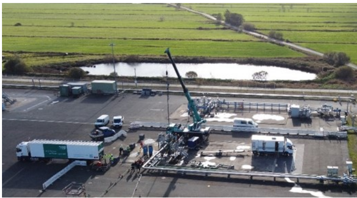
Injection of hydrogen into the borehole of the H2CAST project cavern in Nov. 2022 (Source: H2CAST Etzel)
