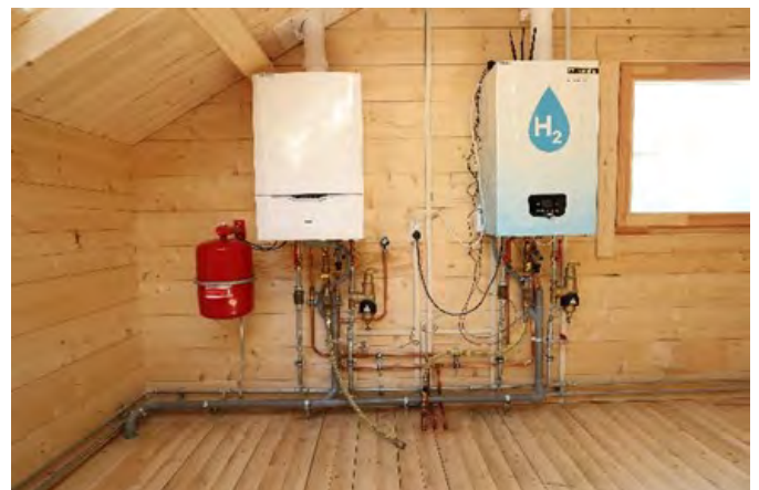
INSIDE THE DEMOS SITE; SOURCE: KIWA
