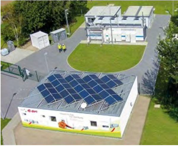
AERIAL PICTURE OF THE WINDGAS FACILITY HAMBURG-REITBROOK | GREGOR SZIELASKO, 2015
