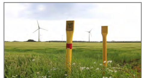
POWER-TO-GAS - THE INVISIBILITY OF THE NATURAL GAS GRID (USCHI DREIUCKER - PIXELIO.DE)
