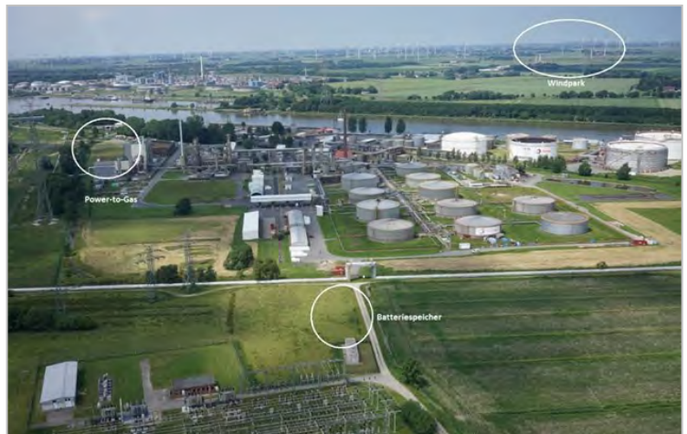
OVERVIEW: POWER-TO-GAS LOCATION BRUNSBÜTTEL (SOURCE: WIND TO GAS ENERGY)
