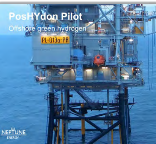
Q13A - A UNIQUE ELECTRIC POWERED PLATFORM (SOURCE: NEPTUNE ENERGY)
