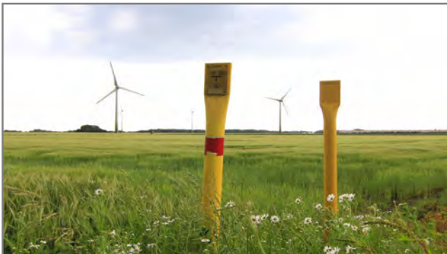
POWER-TO-GAS - THE INVISIBILITY OF THE NATURAL GAS GRID (USCHI DREIUCKER - PIXELIO.DE)
