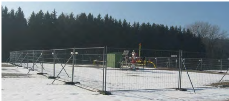
UNDERGROUND SUN STORAGE LEHEN (RAG AUSTRIA)
