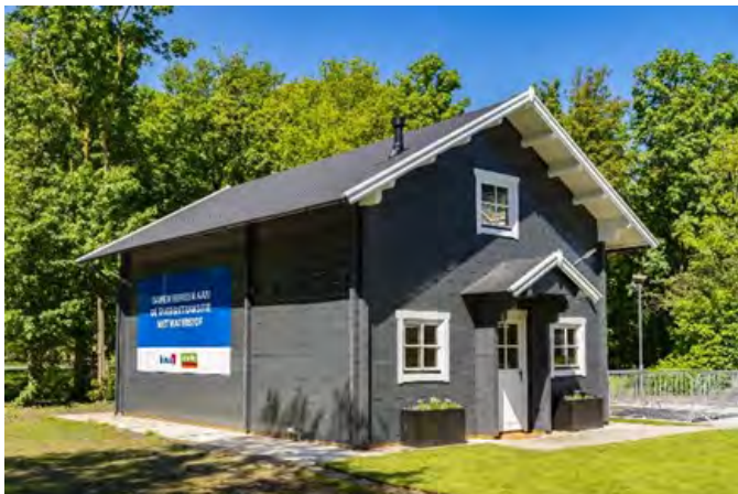
THE HYDROGEN HOUSE; SOURCE: KIWA
