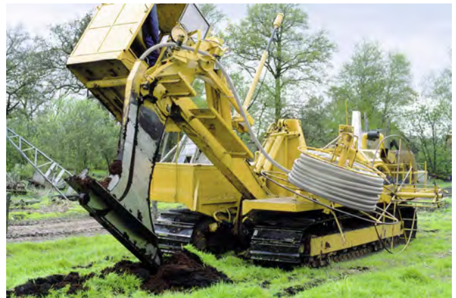
INNOVATIVE TECHNOLOGY - PLOUGHING OF A COMPOSITE PIPING SYSTEM (SOURCE: REHAU)
