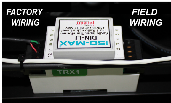
Figure 16: Signal Termination – Swing-Out Rack
