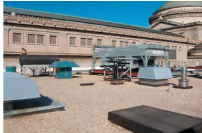
The lean-burn engine's radiator and critical exhaust silencer are roof mounted.
