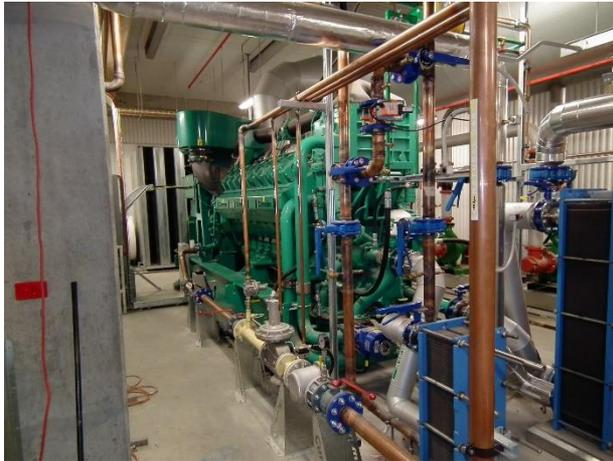
The Cummins Power Generation lean-burn generator set produces up to 1.75 MW of electricity and 4,000 pounds of steam per hour in a CHP application.
