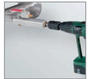
Drill under pressure with the CS drilling jig
