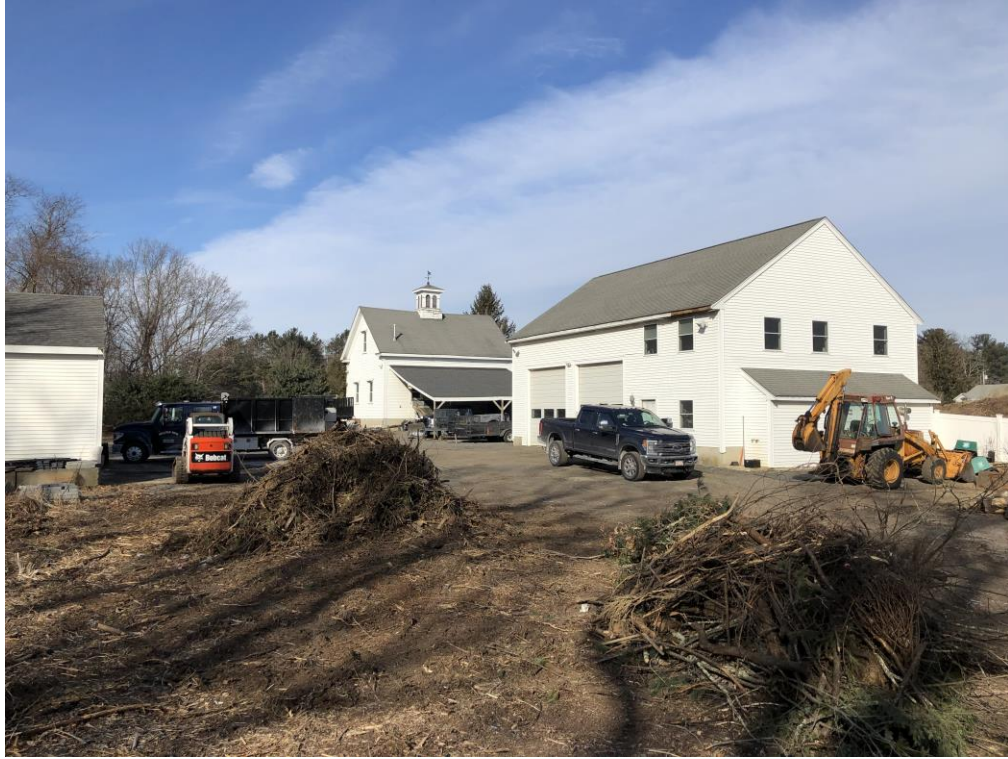
Photo 2 - Degraded area facing West
