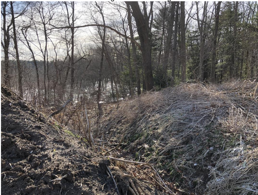
Photo 3 – Degraded area – stockpiles – facing east
