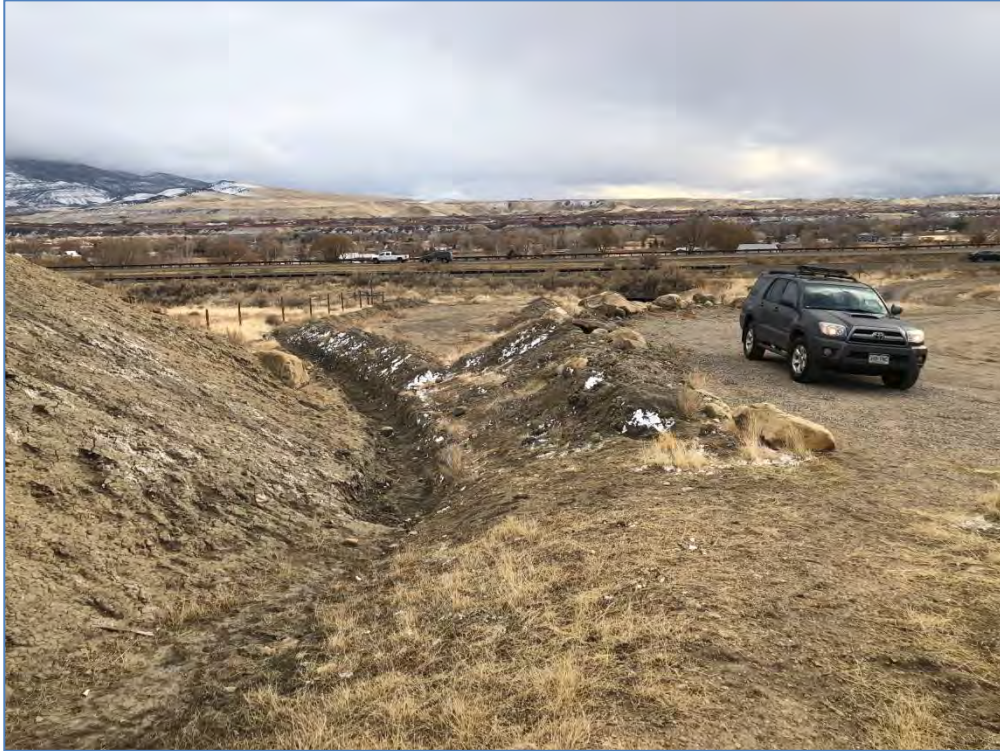
Photo 1: Upstream end of constructed channel.
