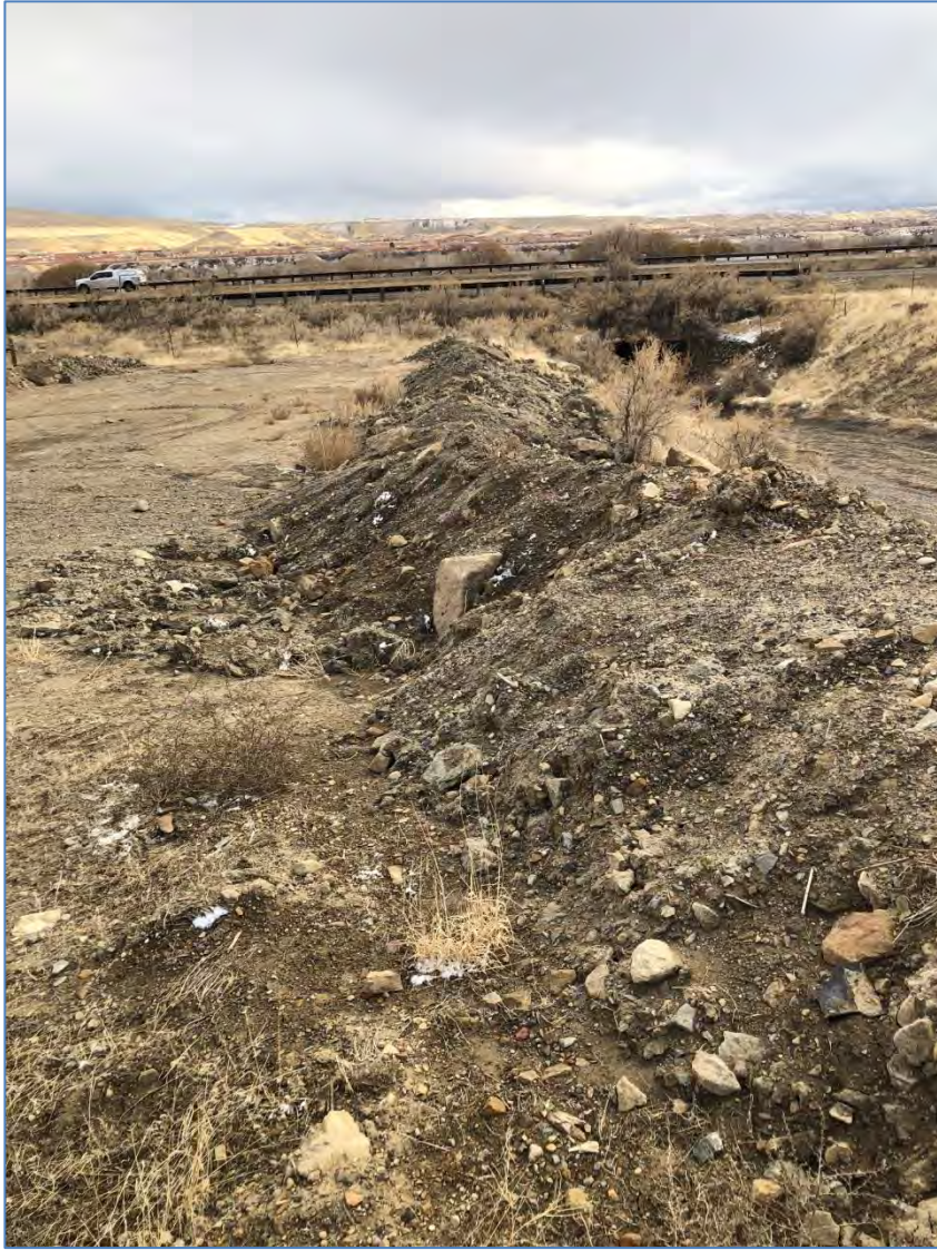
Photo 3: Constructed earthen berm
