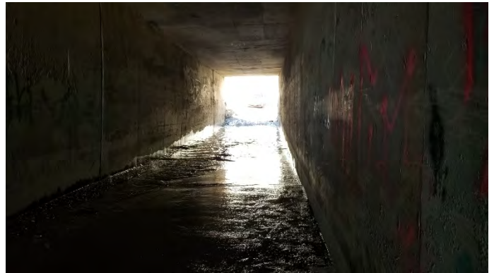
Figure 1 - Existing Culvert: Coal Mine Road Under I-70
