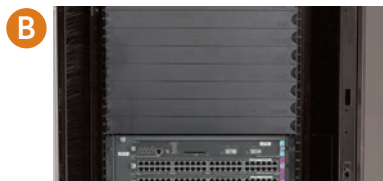
B Blanking panels are available to seal open U spaces.
