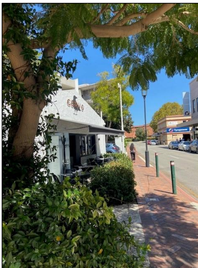
Replacement Awning to 34 St Quentin Avenue, Claremont (view West)
