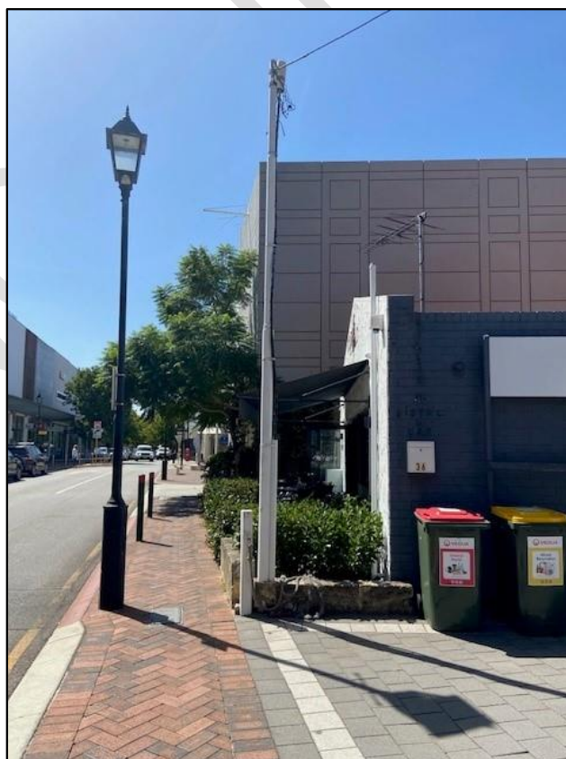
Replacement Awning to 34 St Quentin Avenue, Claremont (view East)
