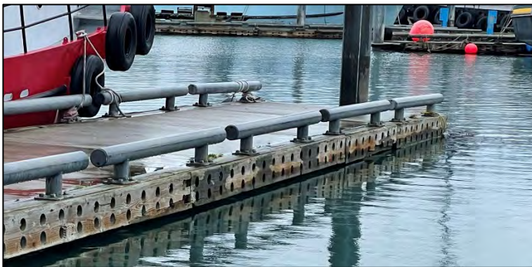
Figure 2.19: Concrete stall float with low freeboard, and in the water at the end.
