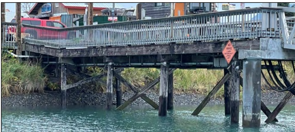
Figure 2.4: Ramp 2 timber pile supported trestle.
