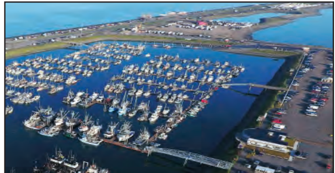
System 4 floats to be replaced.
