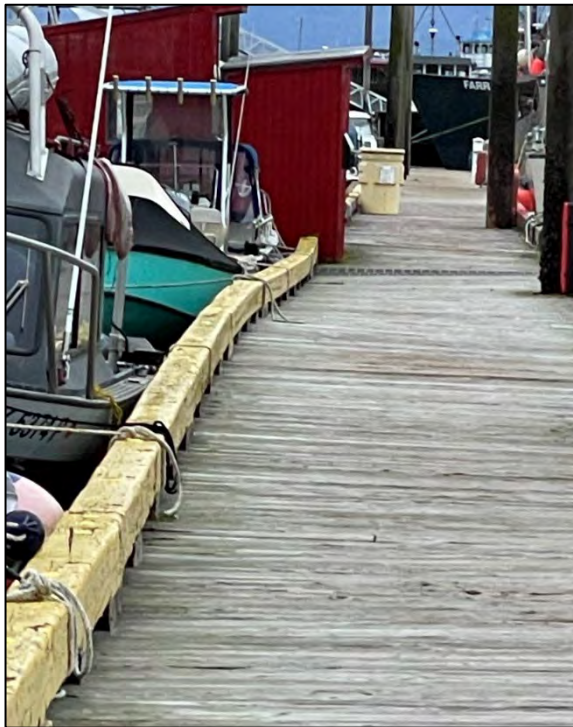
Figure 2.51: Headwalk Float AAA between EE and GG Floats.
