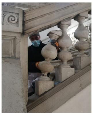
FIG. 4 Desalination of the intermediate landings
