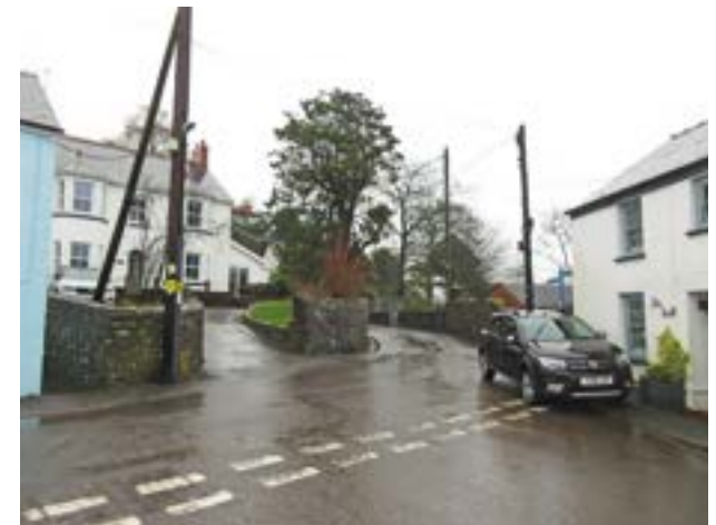
overhead power lines Victoria Street
