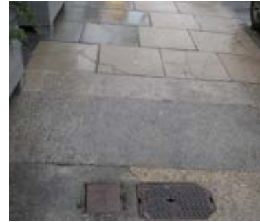
concrete and tarmac paving, King Street
