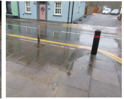
precast concrete paving and a variety of bollards. King Street
