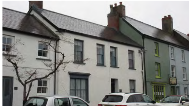
2-3 storey properties on King Street
