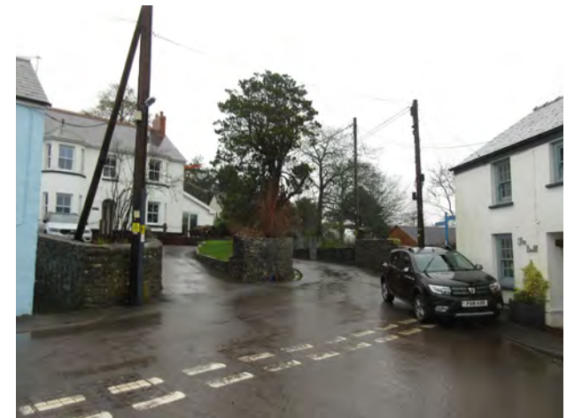
overhead power lines Victoria Street
