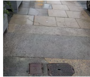
concrete and tarmac paving, King Street
