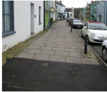
patched mix of low quality surfaces, King Street
