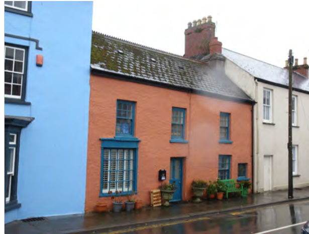
Former shop, Redford House, King Street
