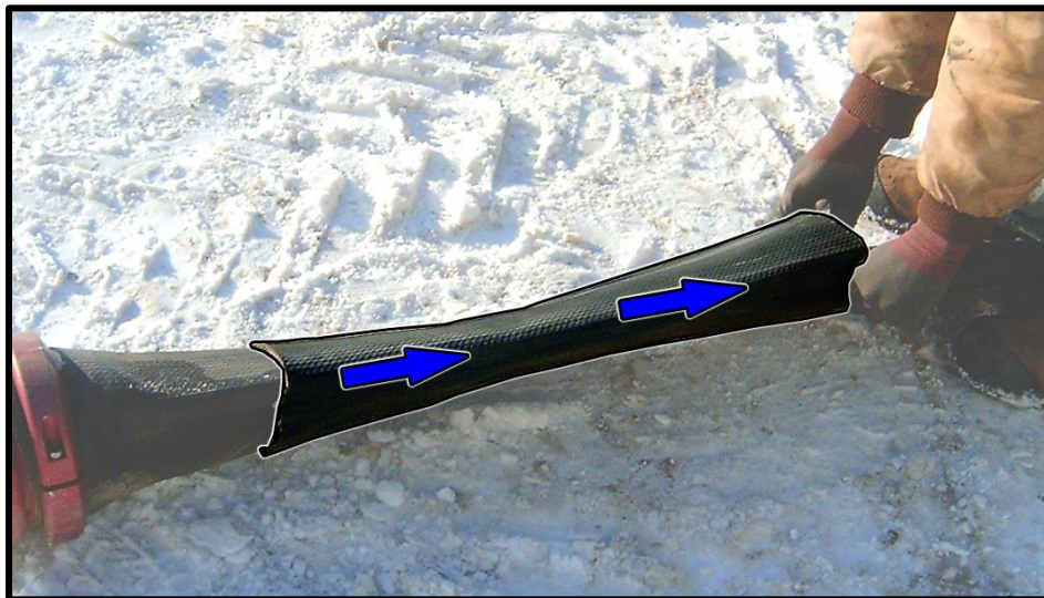
Figure 47 - Pull Repair Sleeve
