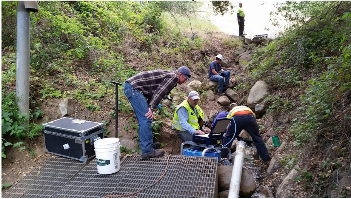
Camera Inspection of Ortega Reservoir Underdrain
