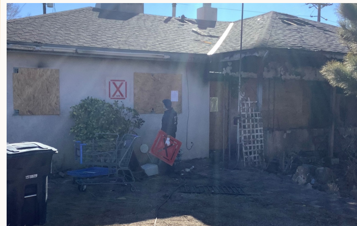
Inspector Horner identifying 9608 Snow Heights as an unsafe building.
