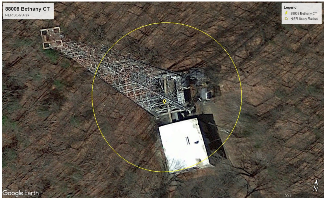
Aerial View of Site
