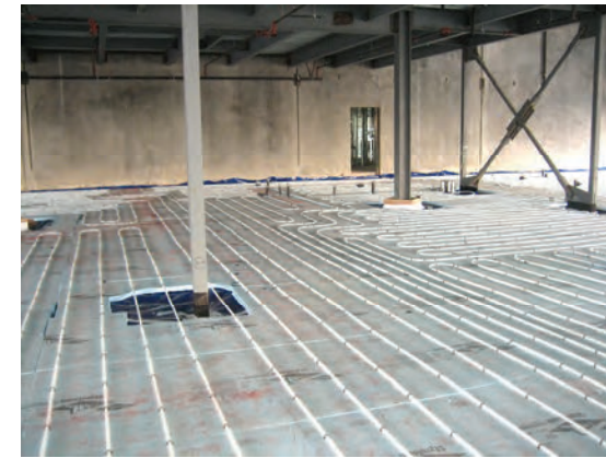
Radiant floor system
