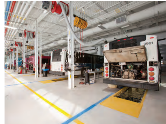
Daylighting - Repair bays
