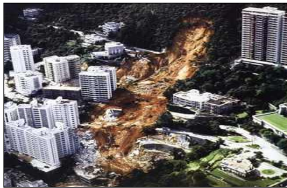
Figure 4. Hong Kong, Po-Shan Road landslide in 1972, presenting the danger of unstable ground conditions, (Photo by Geotechnical Control Office, Hong Kong Government), (Schuster & Highland, 2007).
