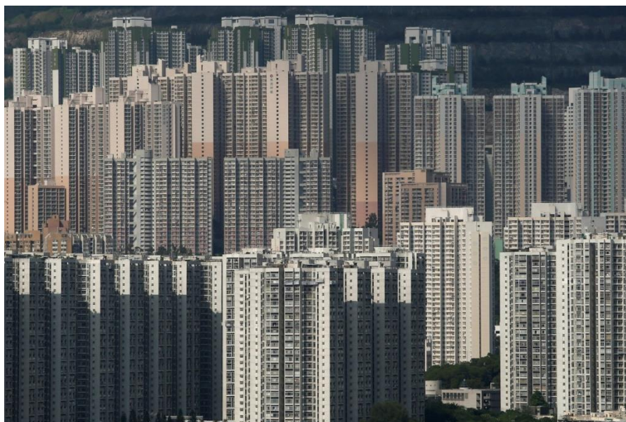
Fig. 10 Housing in Hong Kong
