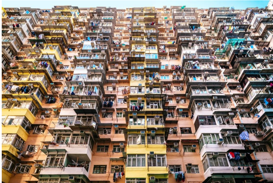
Fig 9. Housing in Hong Kong.
