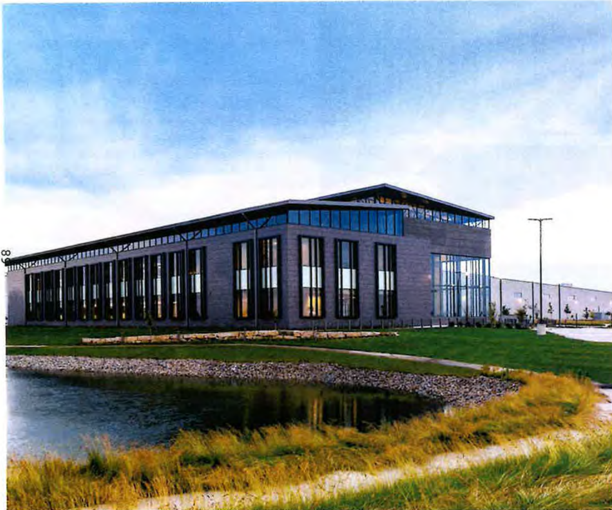
FIGURE 1.09 QUIK TRIP DISTRIBUTION CENTER, BELTON, MISSOURI
