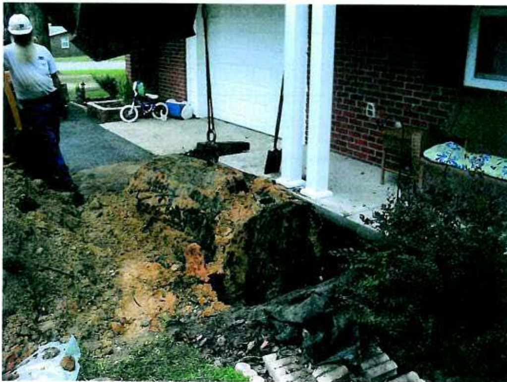
Picture 2: UST 300Ash removal in progress.
