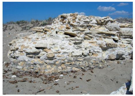
Figure 15. Detail of the opus caementitium of structure H8, from the west. (Forschungsstelle Asia Minor, Münster)
