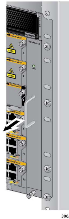
Figure 162. Loosening the AT-SBxFAN12 Fan Module from the Backplane Connector
