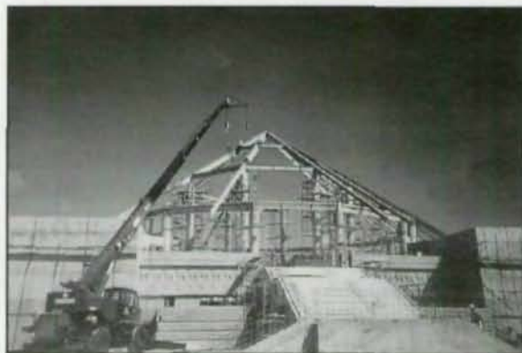
The isometric view and a construction photo reveal the design of the conical-shaped roof of the new Parliament Building.
