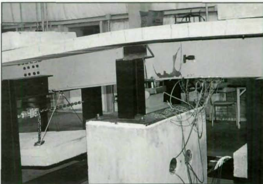
Close up of north interior pier showing large inelastic rotation. Also shown are the lateral bracing, reaction load cell and pin support, and strain gage instrumentation.
