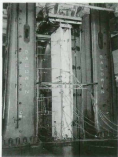
Figure 6 Test Set-up for Beam Column Test (Air bladder on right side of specimen)
