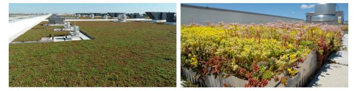
With the green roof on the relocated facility, FedEx is reporting a 30 percent cost savings for energy use (heating and cooling), as compared to the previous facility. Green roofs reduce the heating and cooling demand for facilities and decrease the overall Urban Heat Island Effect of the Airport.
