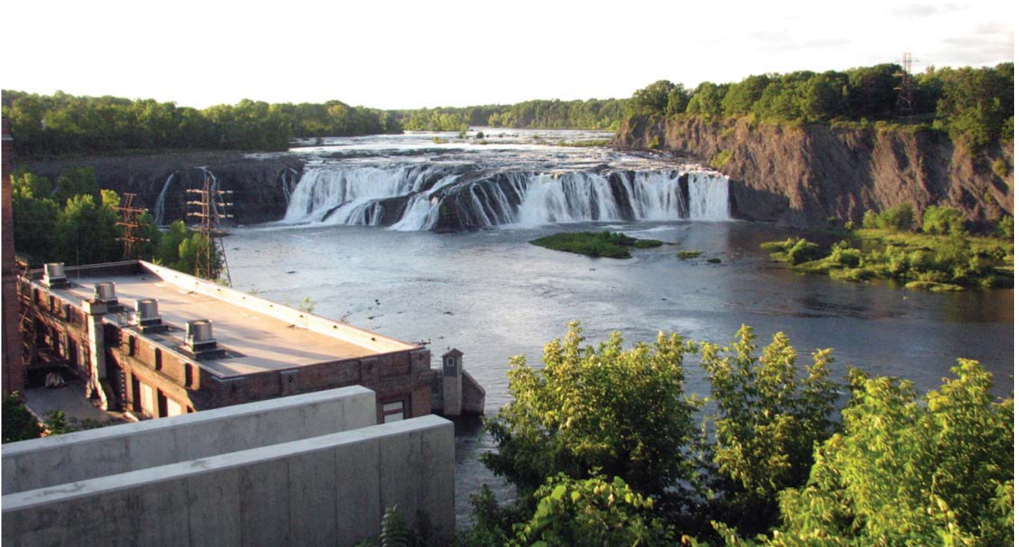
School Street Hydroelectric Power Plant. Located on the scenic Cohoes Falls along the Mohawk River, this facility has a nameplate capacity of 42 MW, and all electricity generated flows into the State's electrical grid. Photo credit: Wikimedia.
