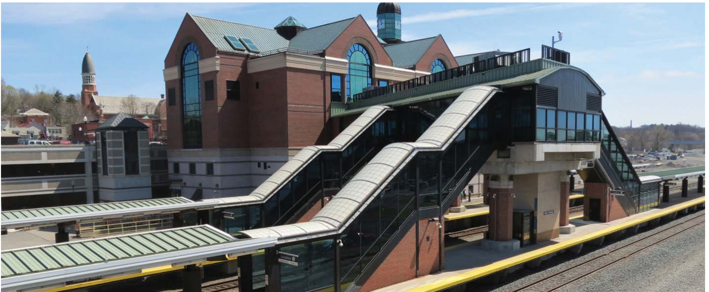
Albany-Rensselaer Train Station. Photo credit: Wikipedia
