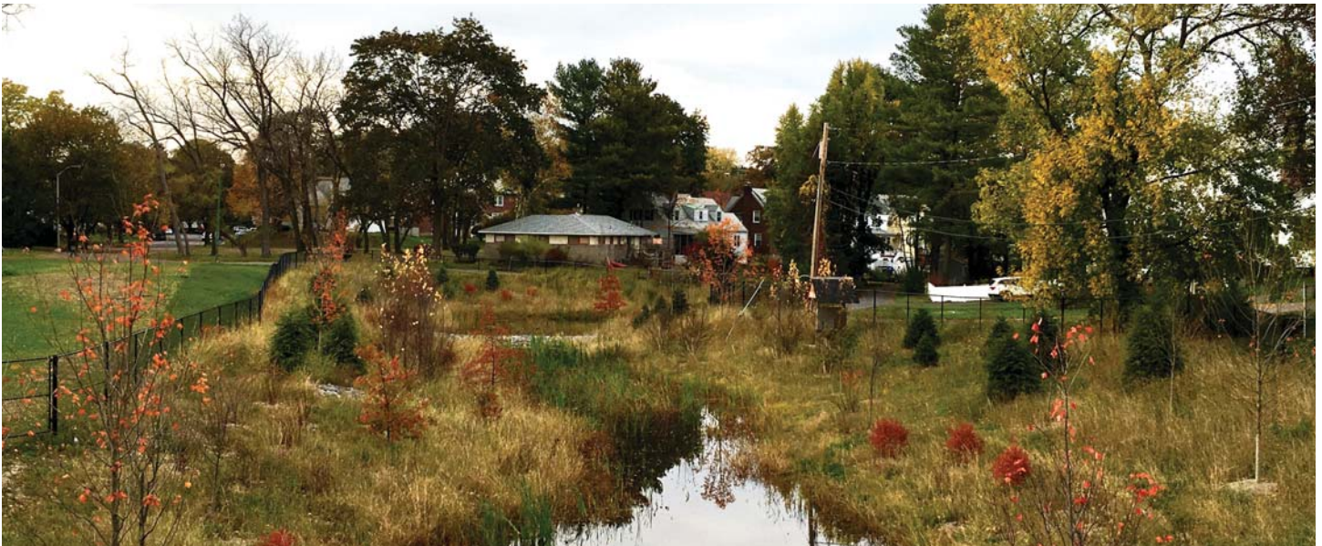
Green Infrastructure. A recently constructed wetland in a residential neighborhood in the City of Albany provides residents with flood mitigation, filters water prior to discharge, reduces strain on the City's sewer system during heavy rain events, and creates new habitat. Photo credit: Bergmann
