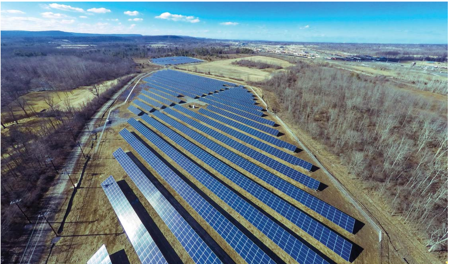
Solar Arrays in Albany County. The top image shows the Capital Region Community Solar Garden in Altamont, which came online in April 2019. The bottom image displays the Bethlehem East solar farm, which was developed on a former clay mine site and supplies town facilities with electricity. Photo credits: Solar Industry Magazine (top image); NextEra Energy Resources (bottom image).
