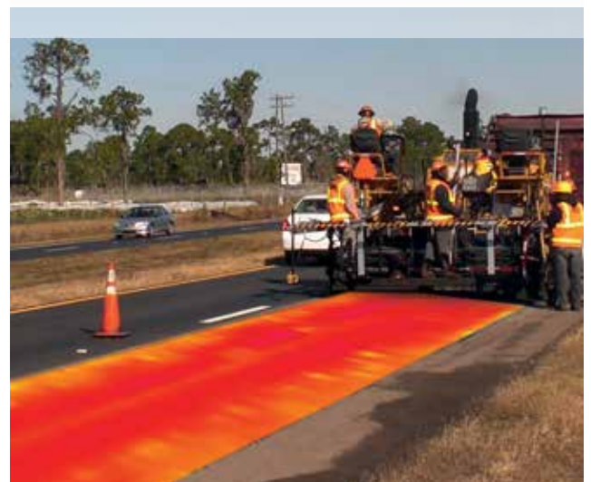
REAL-TIME INFRARED PAVER LEVELING
