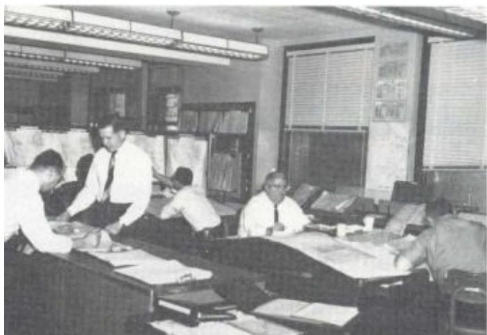
Figure 4-4: Interior of Kansas City Centralized (Terminal) Forecast Facility showing, left to right in foreground, SMSgt Frank Brzeczek, Lt Col James Bunce, Lt Col Robert Miller, and Maj Neil Gardner. In background CMSgt Claborn Gibson, and 1Lt Douglas Fenn.
