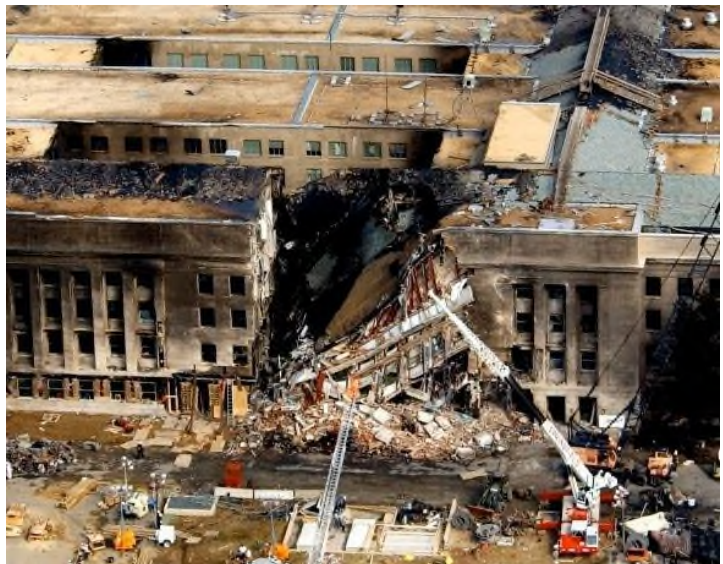
Figure 8-6: Pentagon damage from 11 Sep 2001 Terrorist Attack
