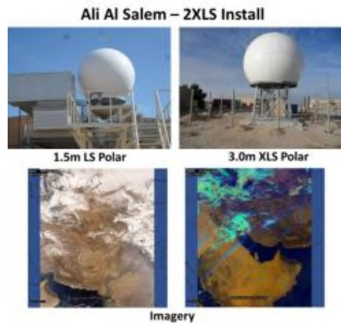
Figure 9-19: MARK IV-B installation and direct readout imagery of SWA at Ali Al Salem AB, Kuwait
