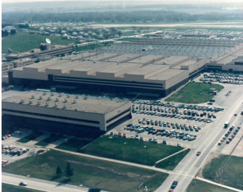
Figure 8-1: Martin Bomber Building (Bldg D) Offutt AFB, NE--home of newly formed Air Force Weather Agency. The smaller building was the Frady Fitness Center, It was demolished several years later.
