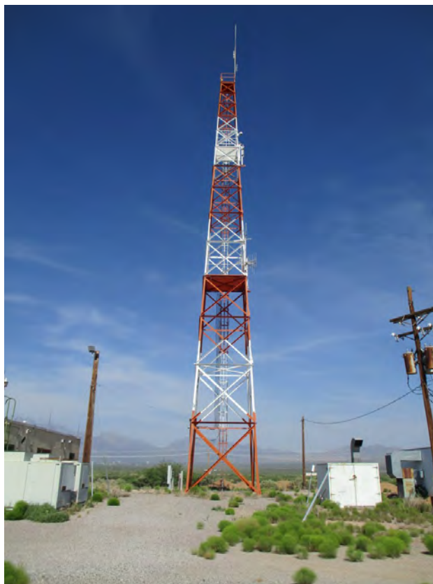
Figure 182. Property 20711 Radio Tower, view to the west.
