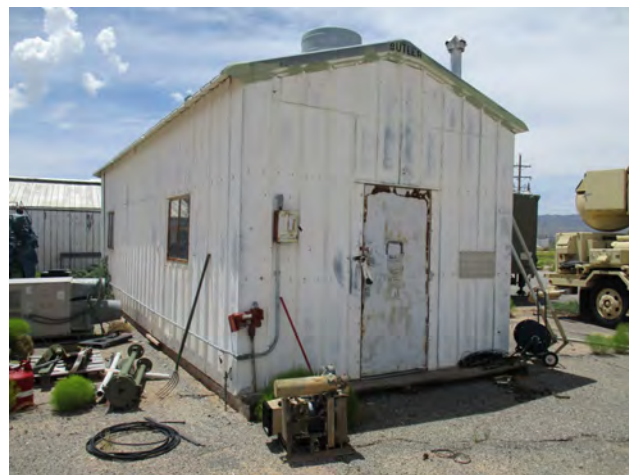
Figure 163. Property H3057, east and south elevations, view to the northwest.
