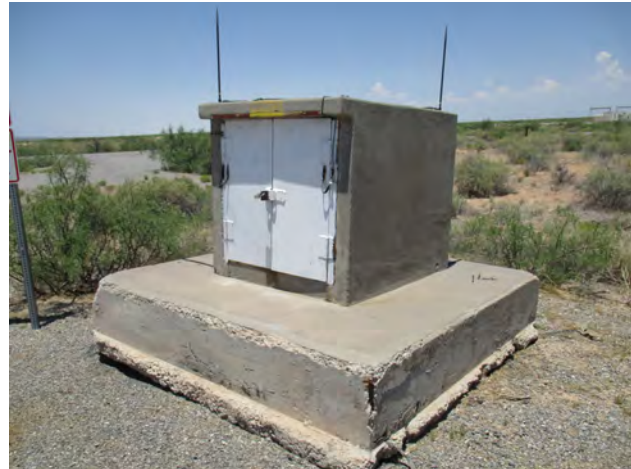
Figure 138. Property 34933, south and west elevations, view to the northeast.
