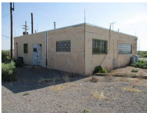
Figure 180. Property 20710, south and west elevations, view to the northeast.
