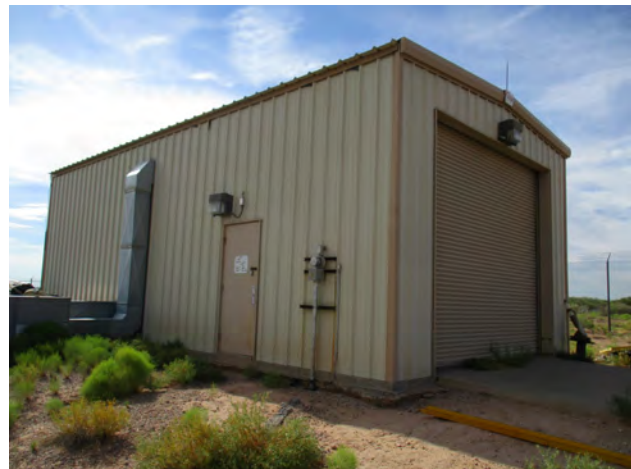
Figure 173. Unknown Pre-manufactured Building 1, north and west elevations, view to the southeast.
