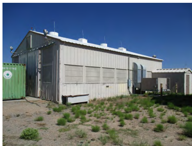
Figure 71. Property 20540, south and east elevations, view to the northwest.
