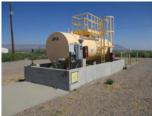
Figure 142. Property 20767, south and east elevations, view to the northwest.
