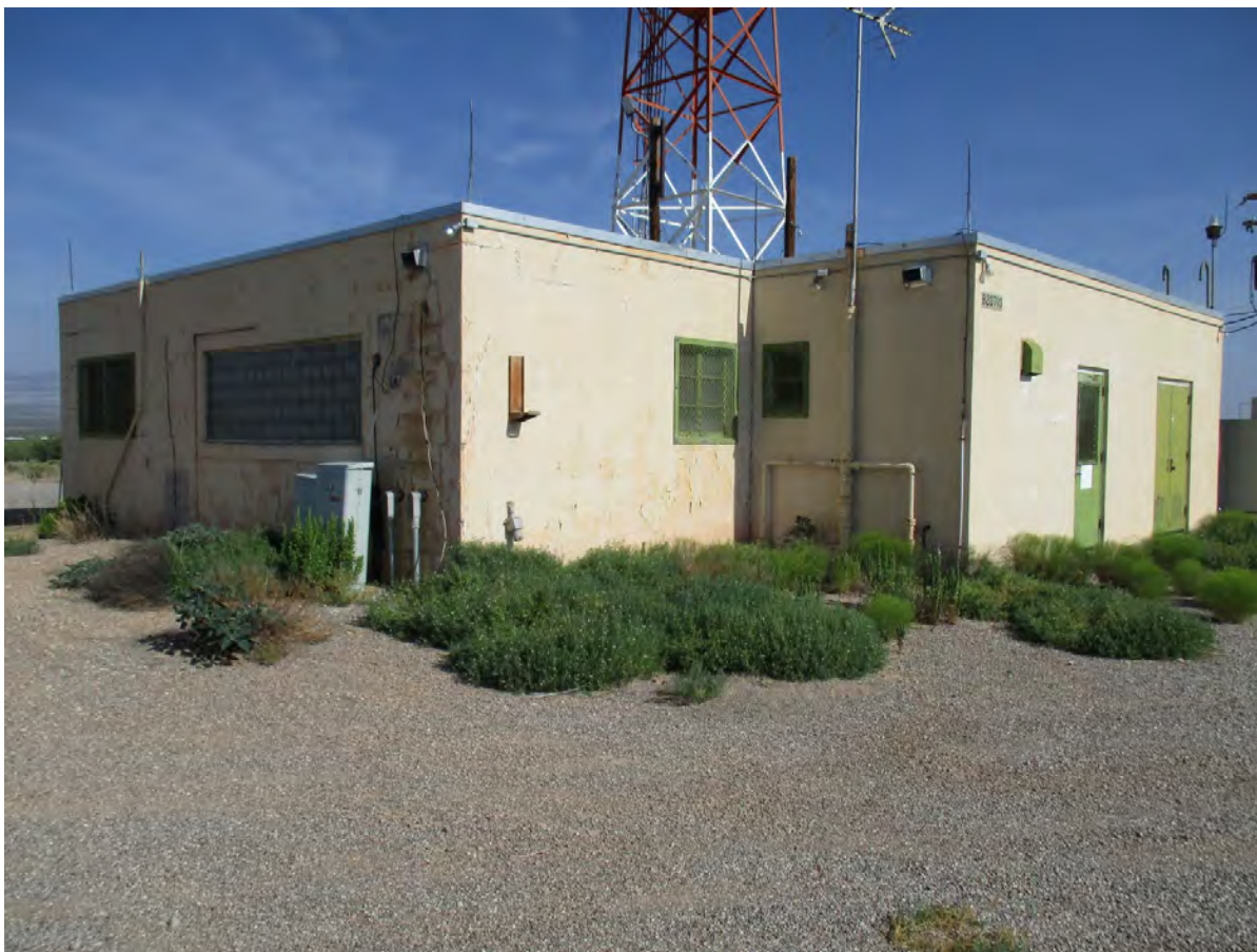
Figure 178. Property 20710, east and south elevations, view to the northwest.
