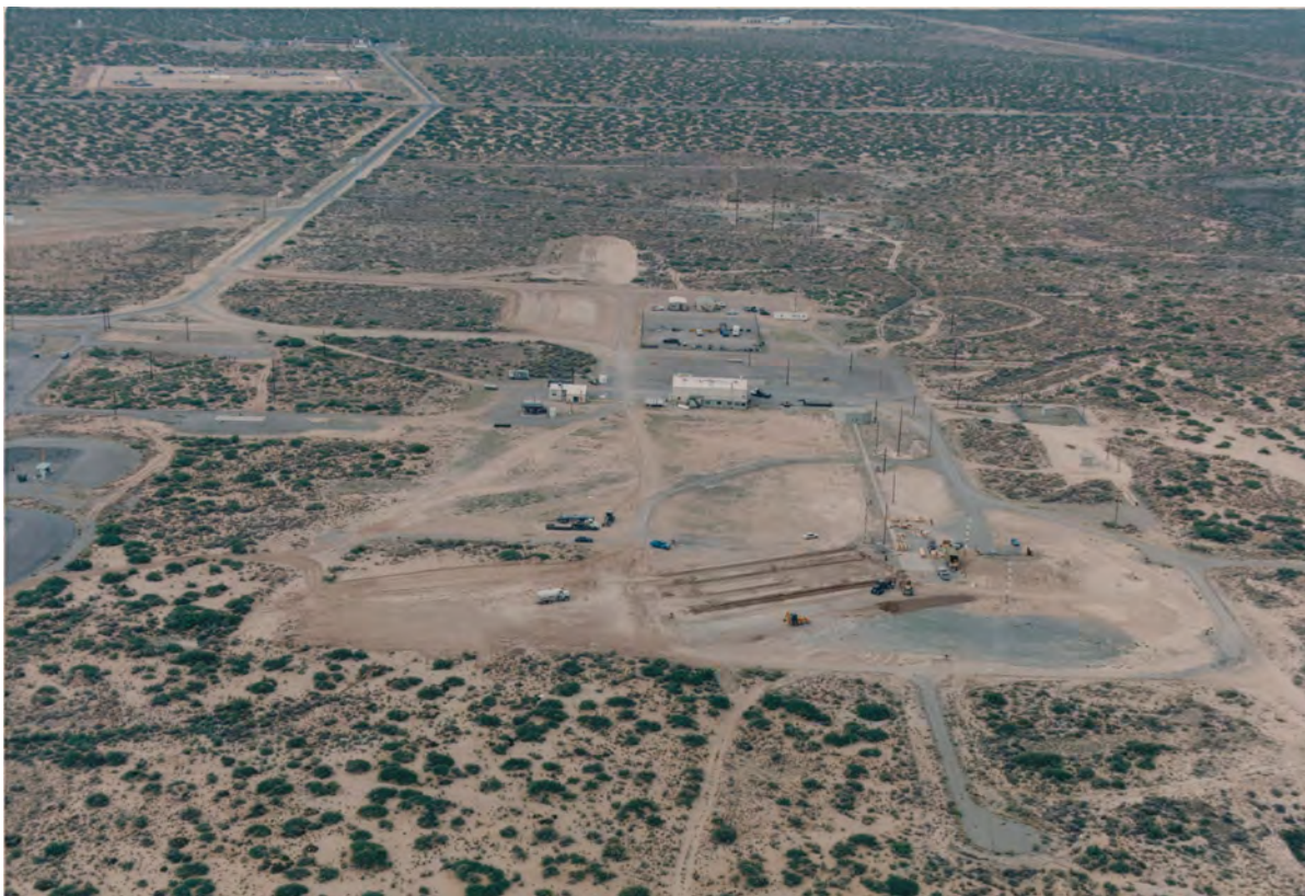
Figure 56. Hera launch pad and shelter under construction at LC-32 in 1994 ( courtesy WSMR Museum Archives ).
