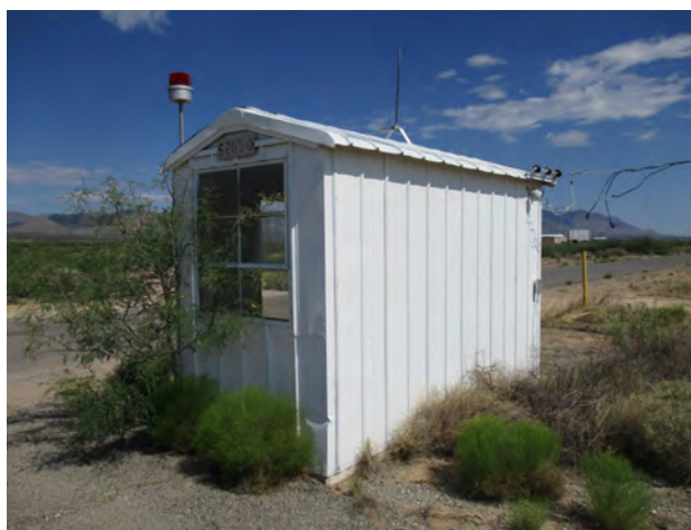
Figure 198. Property 20510 Guard House, south and east elevations, view to the northwest.
