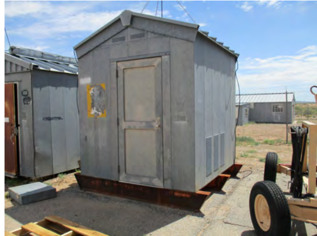
Figure 170. Unknown Portable Building 2, west and south elevations, view to the northeast.
