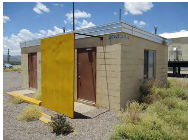
Figure 113. Property 20506, south and east elevations, view to the northwest.
