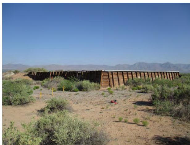
Figure 75. Property 20533, south and east sides, view to the northwest.
