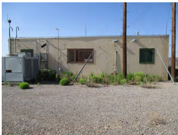
Figure 181. Property 20710, north elevation, view to the south.
