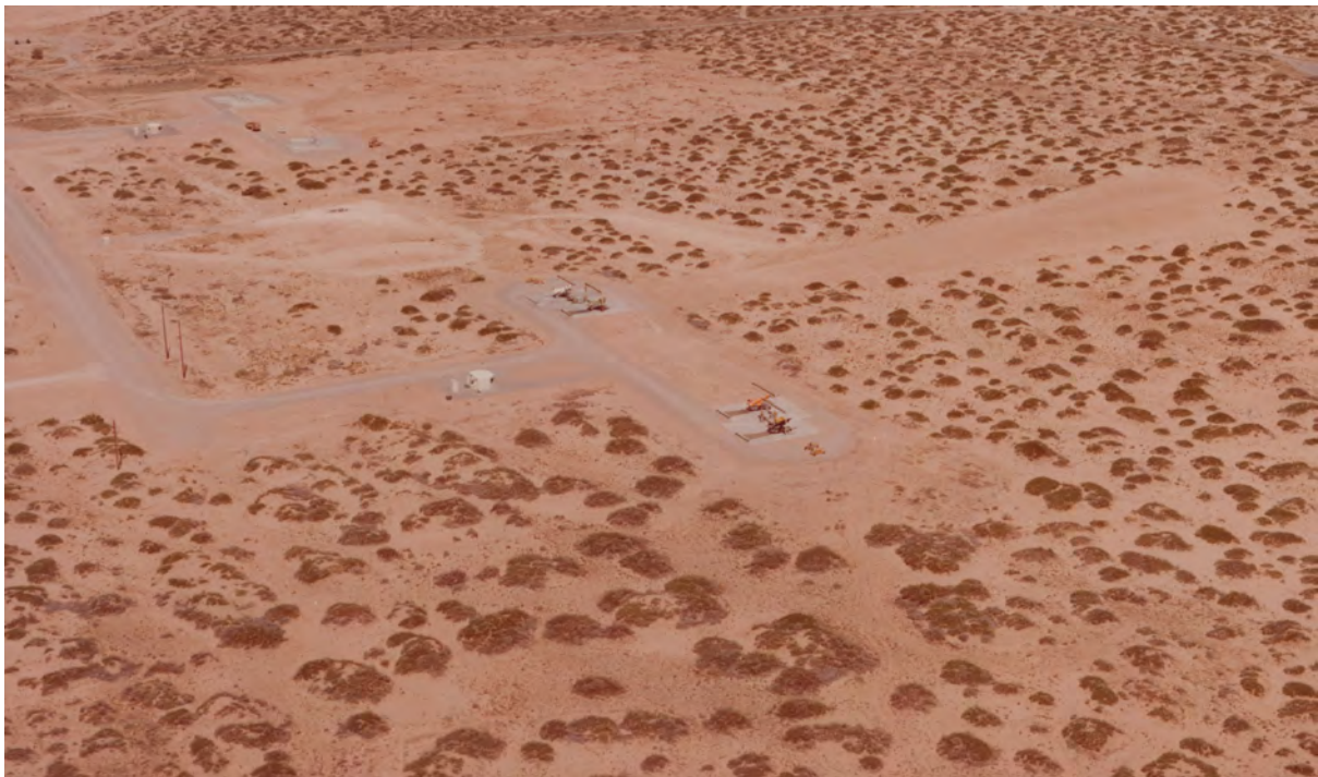
Figure 51. Aerial overview of the MTLC at LC-32, view to the northwest ( photo courtesy WSMR Museum Archives ).
