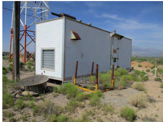
Figure 187. Property 20710A, north and east elevations, view to the southwest.
