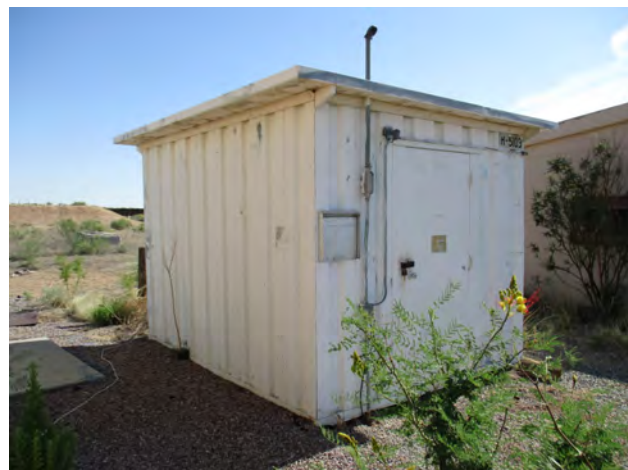
Figure 78. Property H5103, south and west elevations, view to the northeast.
