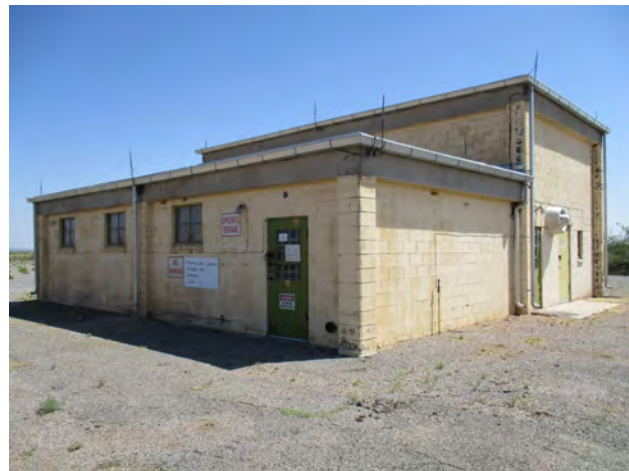
Figure 133. Property 20746, west and south elevations, view to the northeast.
