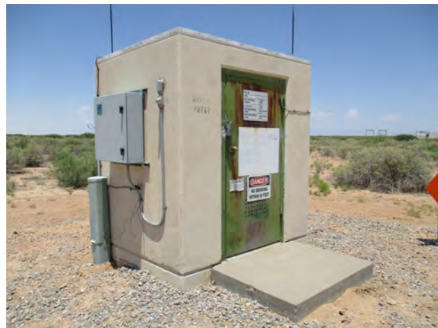
Figure 136. Property 20752, south and west elevations, view to the northeast.
