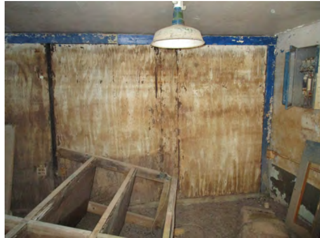
Figure 68. The interior of the Blue Room with boarded over east portion, view to the east.
