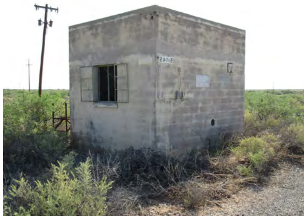
Figure 183. Property 20712, south and west elevations, view to the northeast.
