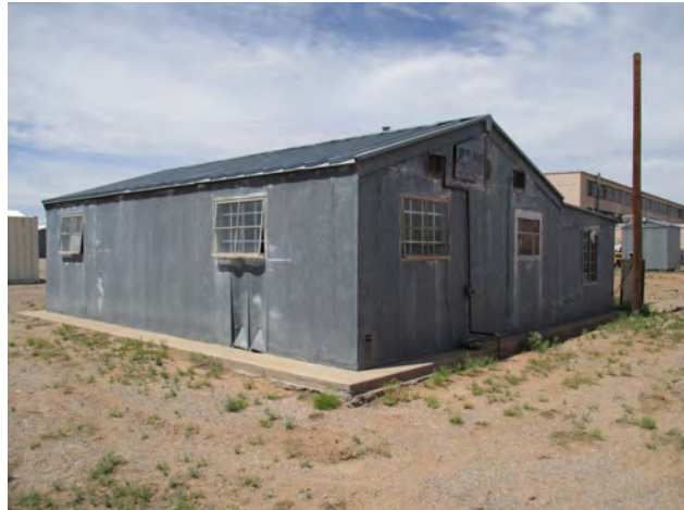
Figure 176. Unknown Pre-manufactured Building 2, east and north elevations, view to the southwest.
