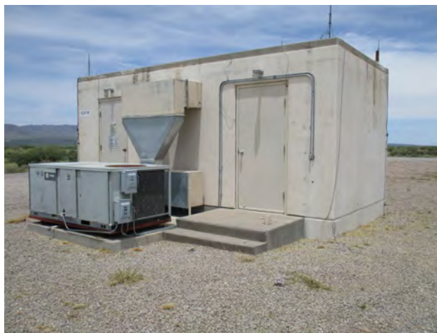
Figure 121. Property 20758, south and east elevations, view to the northwest.
