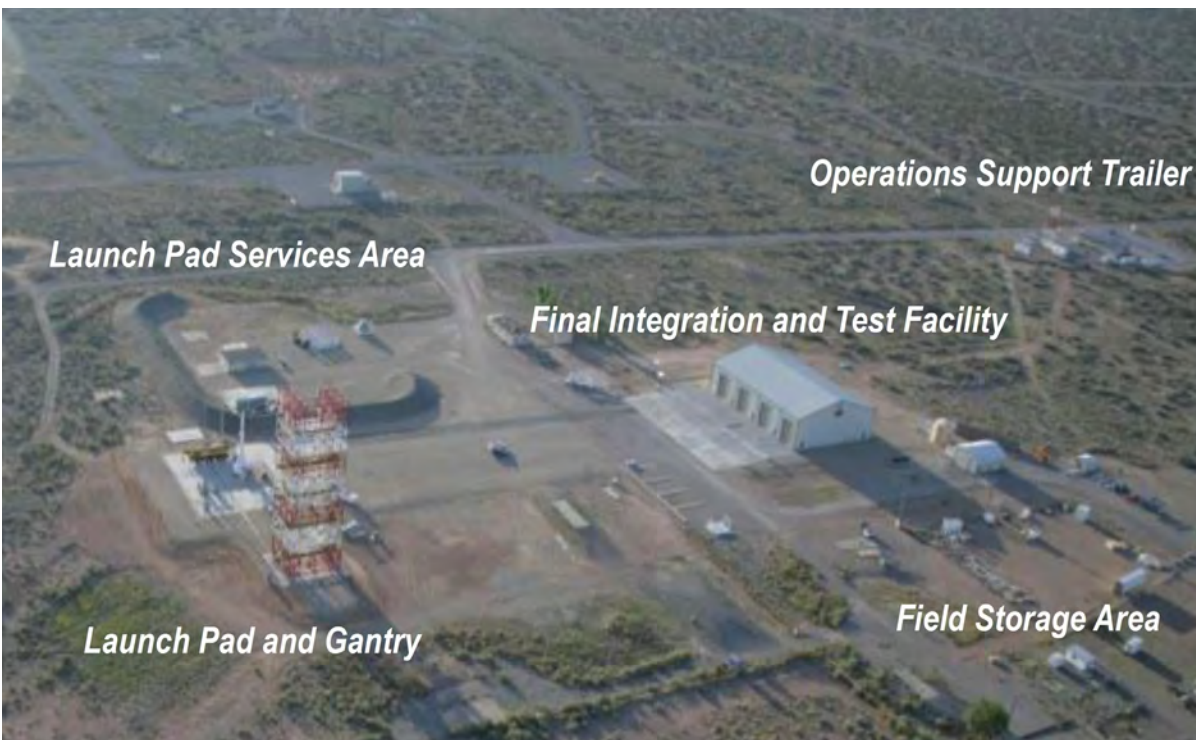
Figure 58. Overview of Orion LAS facilities at LC-32 ( adapted from Hackenburg and Hicks 2007 ).
