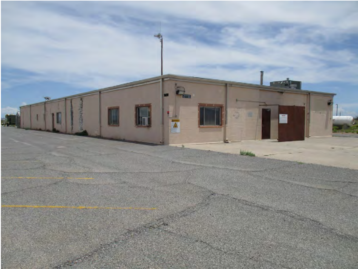
Figure 151. Property 27156, north and east elevations, view to the southeast.
