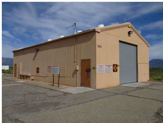
Figure 149. Property 21751, south and east elevations, view to the northwest.
