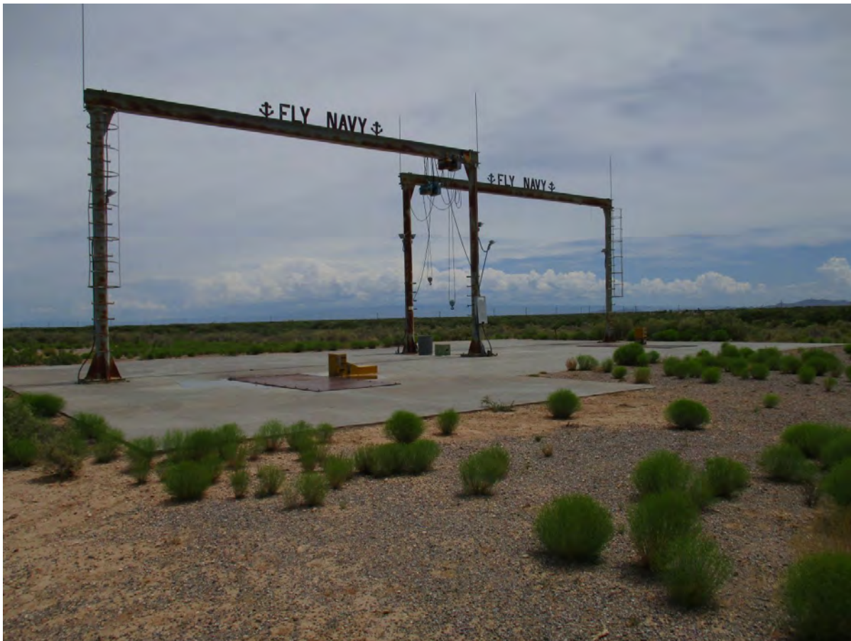
Figure 128. Properties 20769 and 20770 launch pads, view to the northeast.
