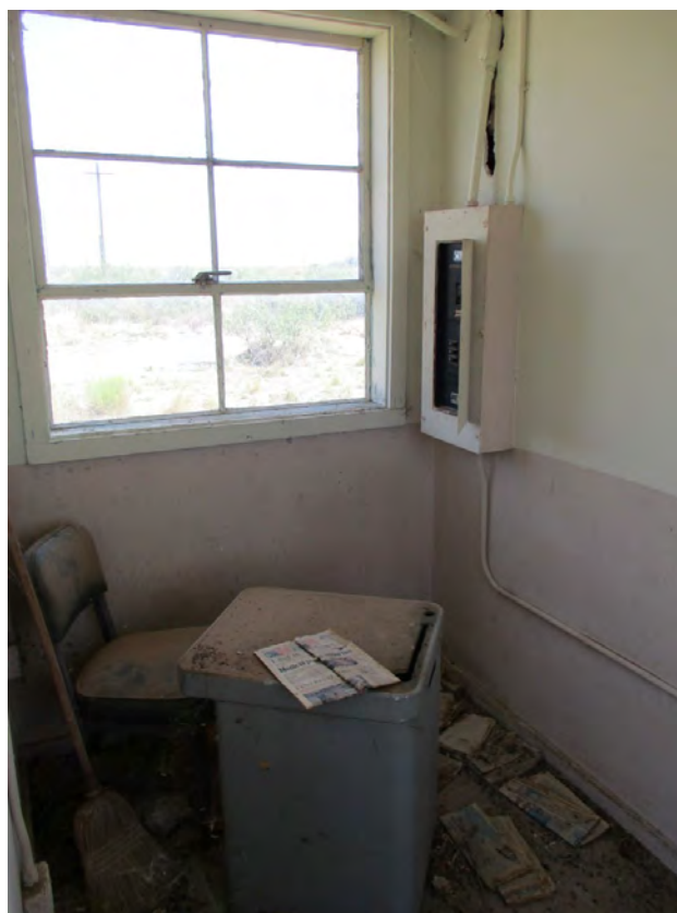
Figure 199. Property 20510, view of interior, view to the north.
