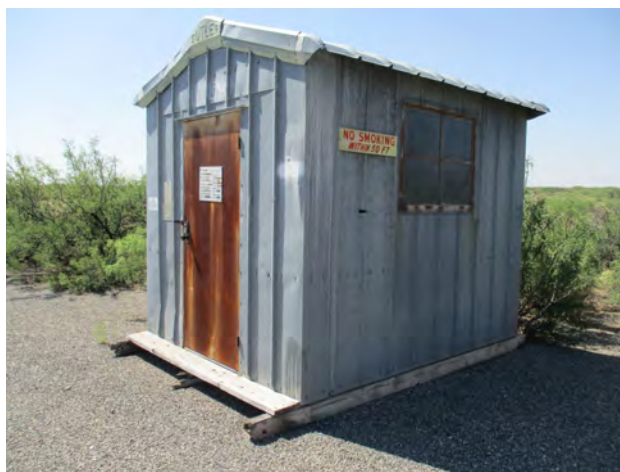
Figure 143. Property H3220, north and west elevations, view to the southeast.
