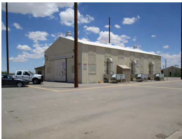
Figure 102. Property 20525, south and west elevations, view to the northeast.
