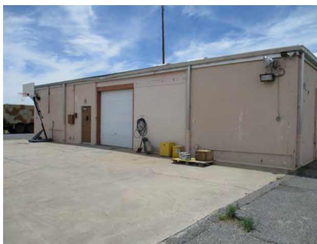
Figure 153. Property 21756, east elevation, view to the southwest.
