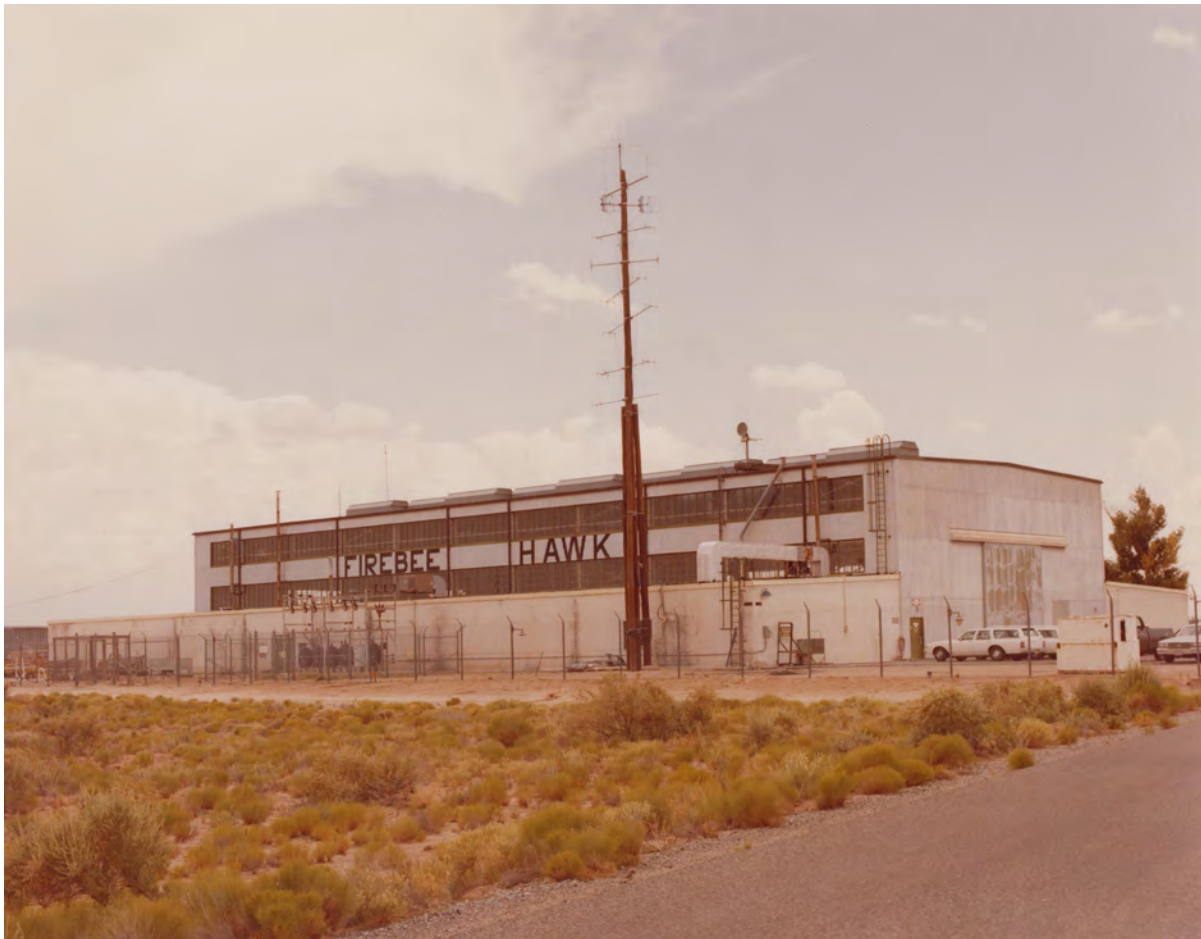
Figure 160. A 1983 photograph of Property 21759, north and west elevations ( WSMR realty files ).
