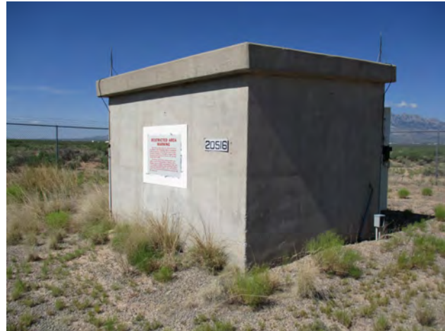
Figure 112. Property 20516, east and north elevations, view to the southwest.
