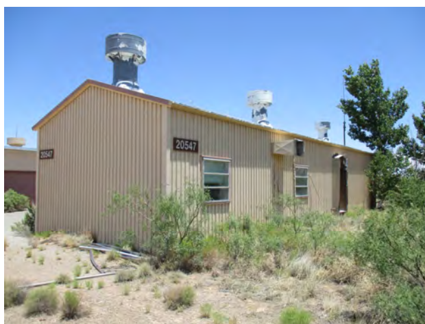
Figure 174. Unknown Pre-manufactured Building 2, south and west elevations, view to the northeast.
