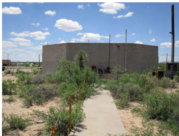
Figure 107. Property 20524 Blast Barricade, north side, view to the south.
