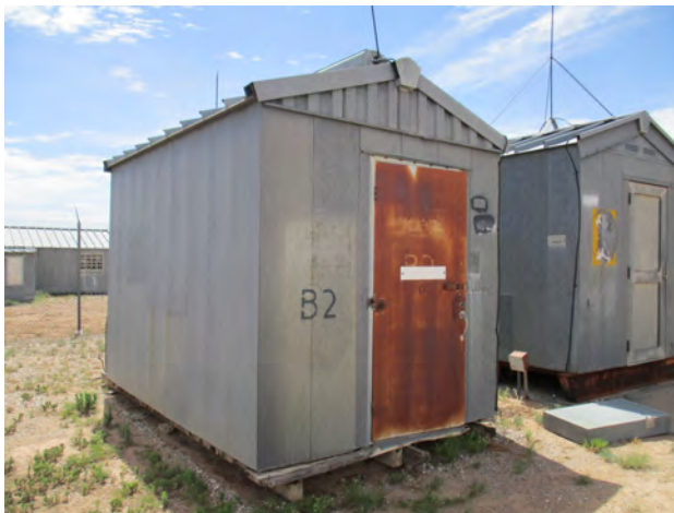
Figure 171. Unknown Portable Building 3, west and north elevations, view to the southeast.
