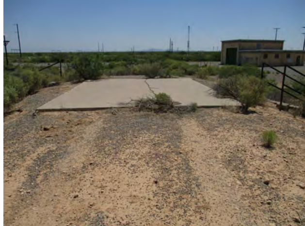
Figure 129. Unknown Instrument Platform 1, concrete foundation on top of mound, view to the southeast.
