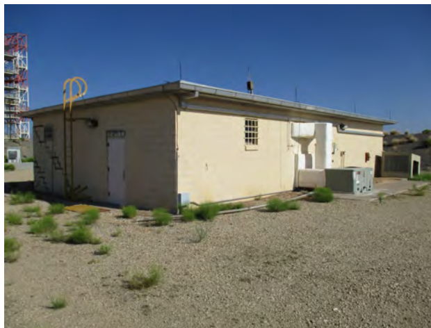
Figure 85. Property 20555, south and east elevations, view to the northwest.
