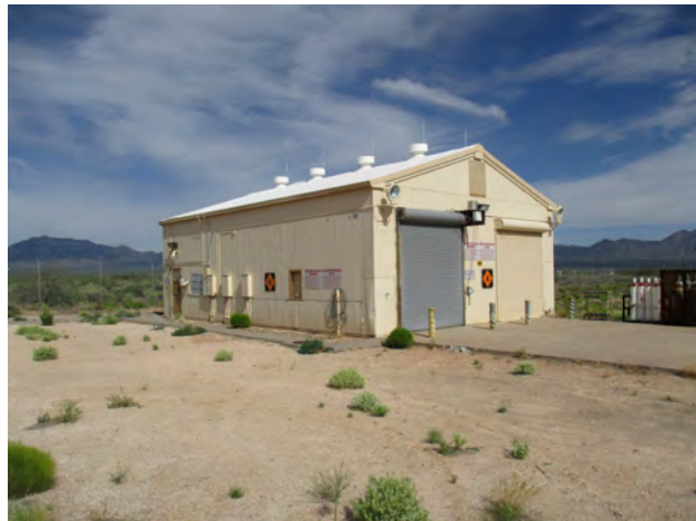
Figure 147. Property 21750, south and east elevations, view to the northwest.
