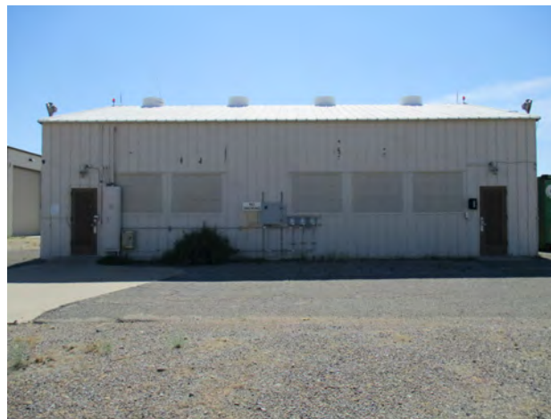
Figure 70. Property 20540, west elevation, view to the east.
