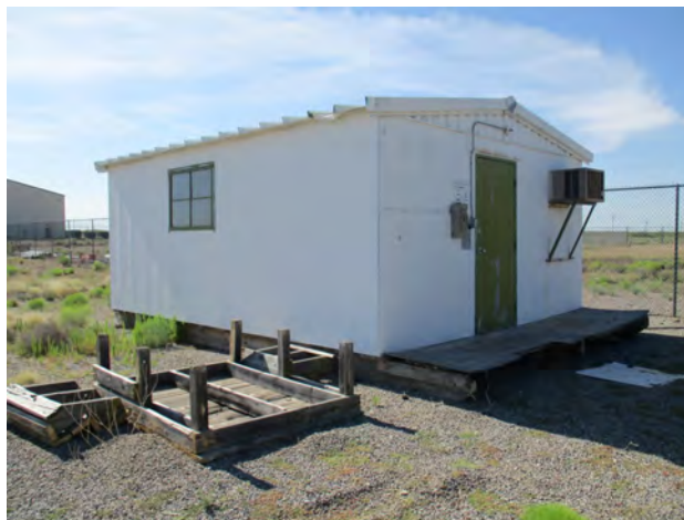
Figure 79. Property WS00910/HS052C, north and west elevations, view to the southeast.
