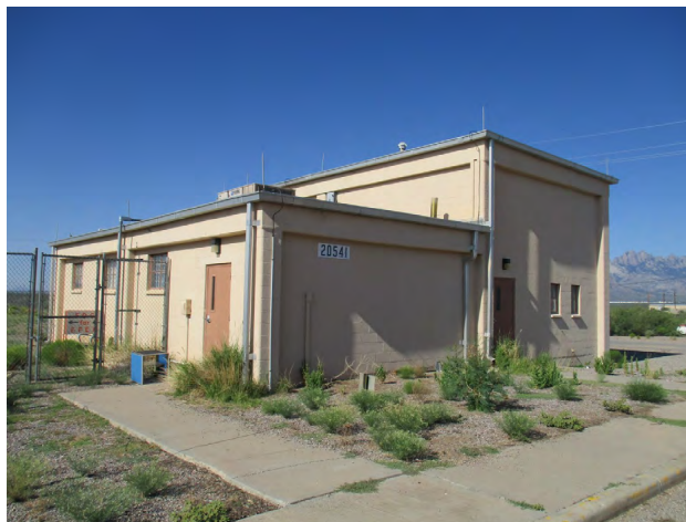
Figure 122. Property 20755, view to the southeast.
