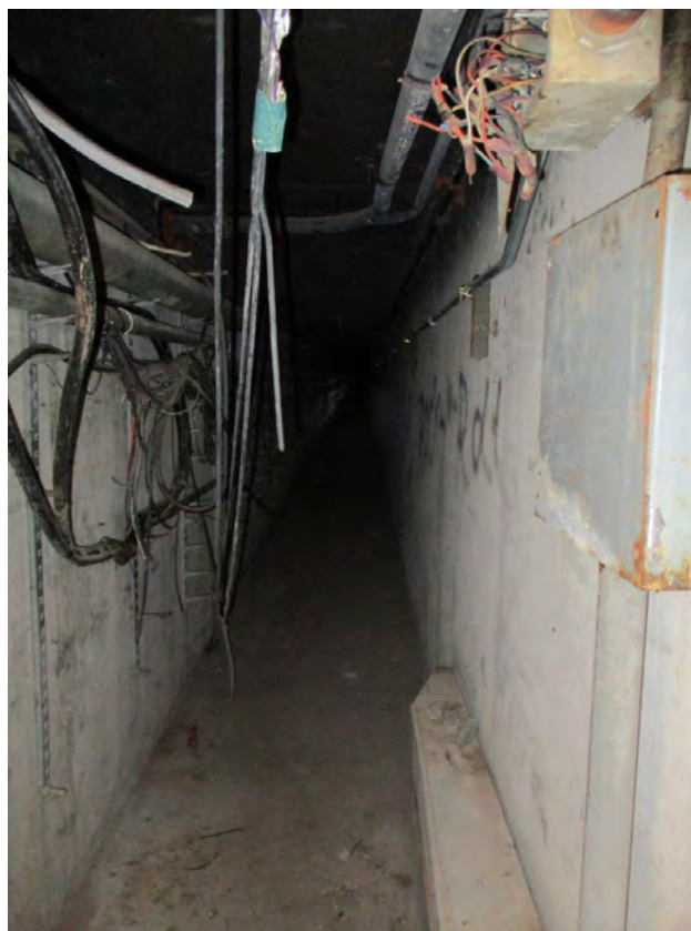
Figure 95. Property 20521, view south down cable tunnel from the electrical vault room.
