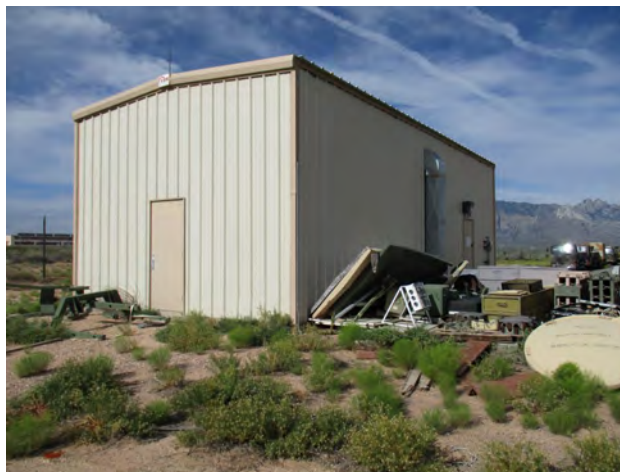
Figure 175. Unknown Pre-manufactured Building 1, east and south elevations, view to the southwest.
