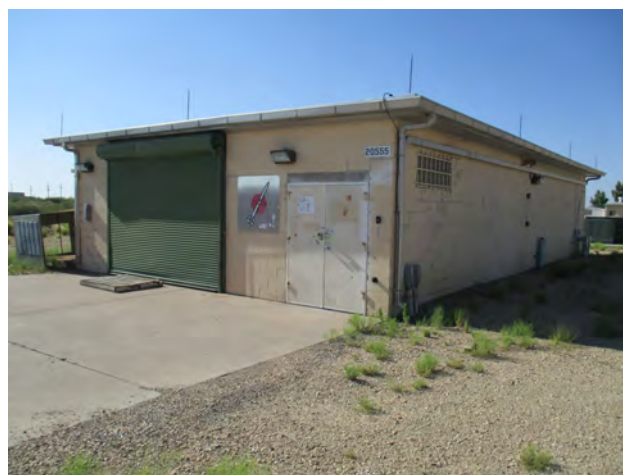
Figure 84. Property 20555, south and west elevations, view to the southeast.
