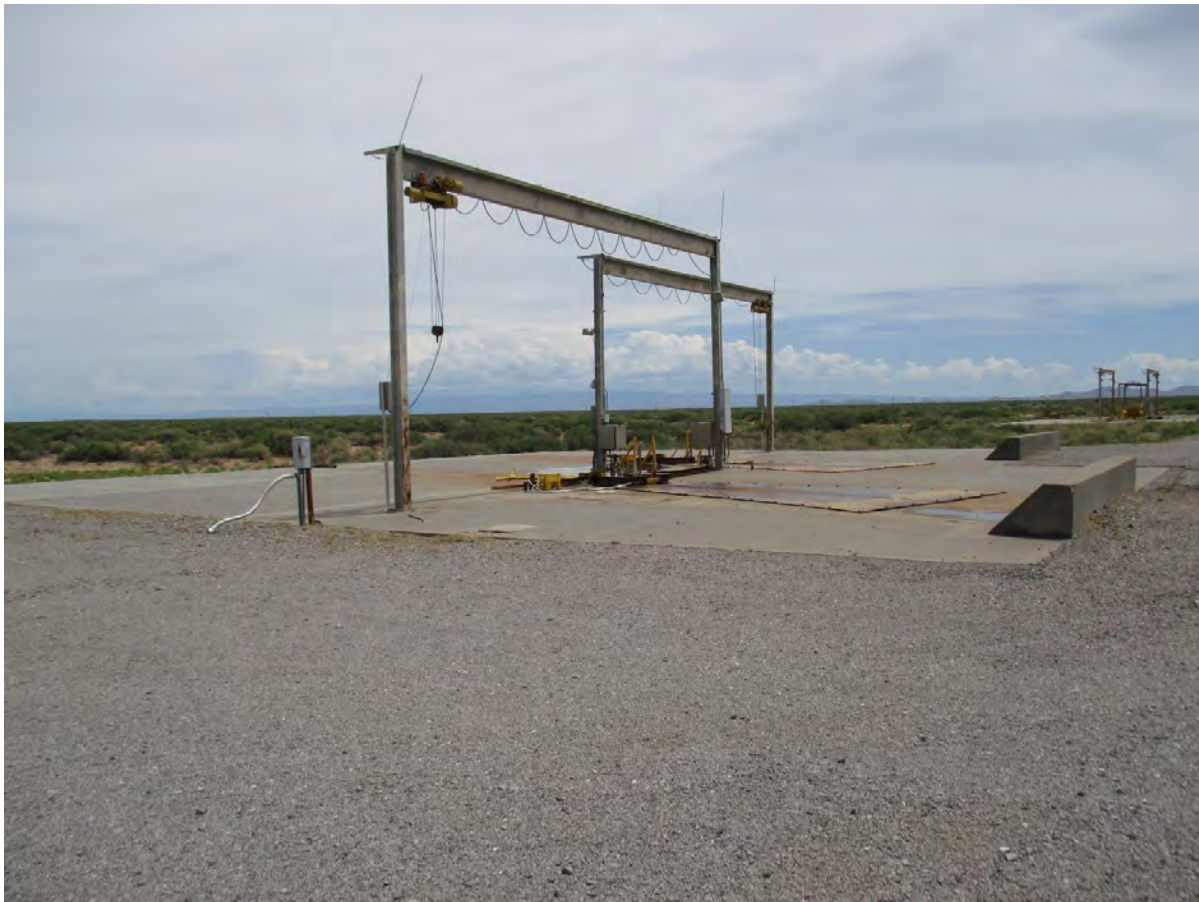
Figure 125. Property 20759 launch pads, view to the northeast.
