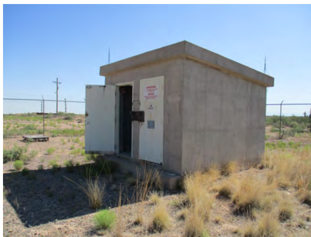
Figure 111. Property 20516, west and south elevations, view to the northeast.
