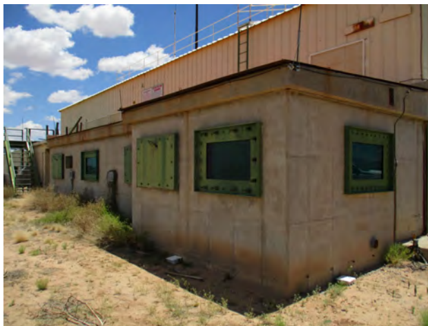
Figure 101. Property 20525, north elevation, view to the southeast.
