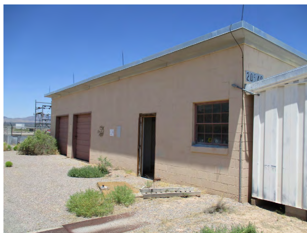
Figure 126. Property 20760 launch pads, view to the northeast.
