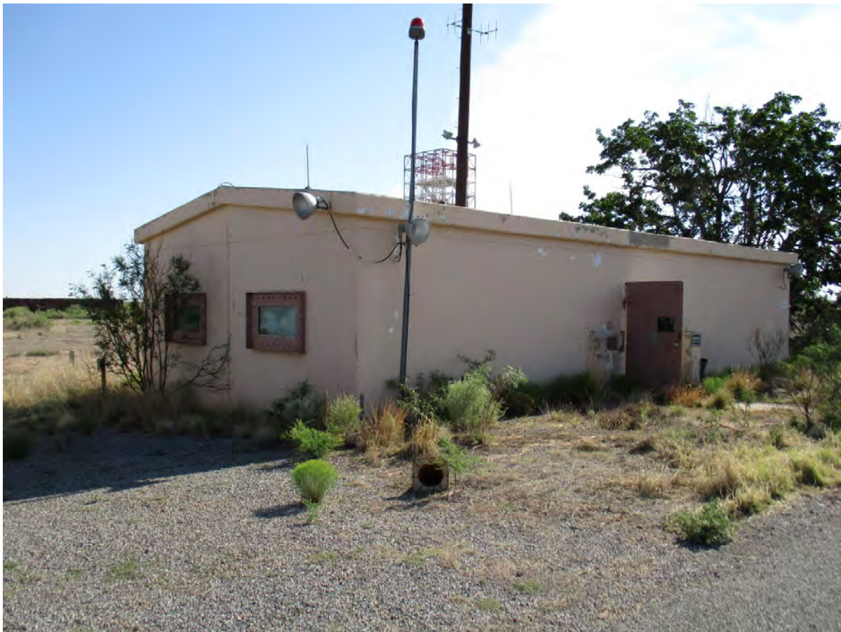
Figure 61. Property 20542, south and west elevations, view to the northeast.
