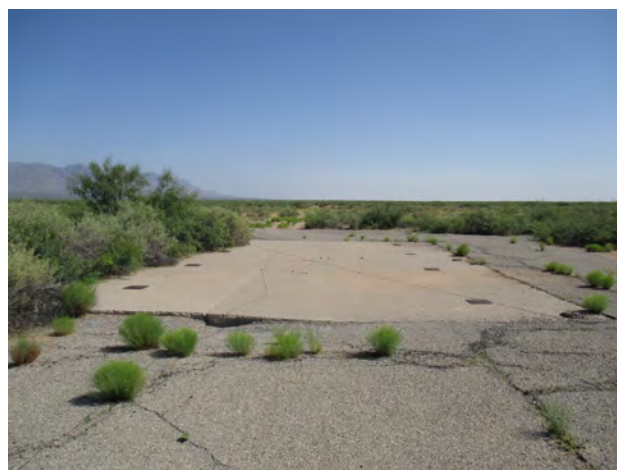
Figure 66. Property 20545 Launch Pad, view to the north.
