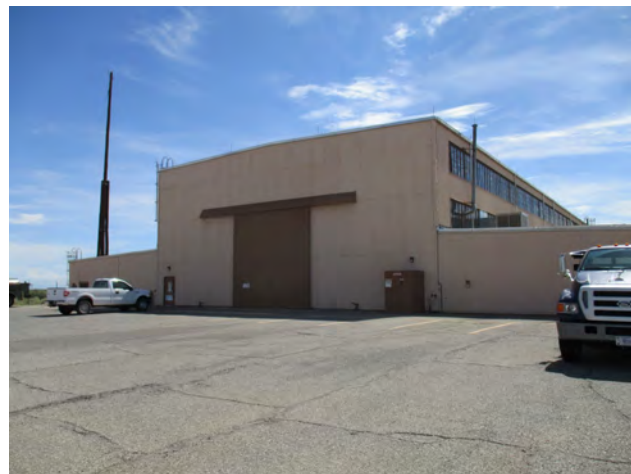
Figure 155. Property 21759, west elevation, view to the northeast.
