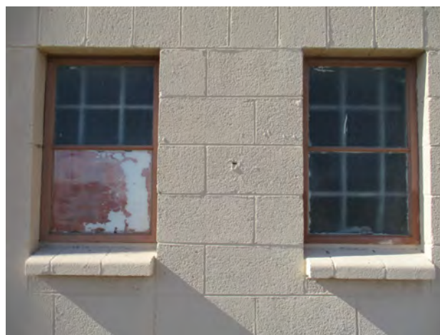
Figure 74. Property 20541, window detail on the west elevation.
