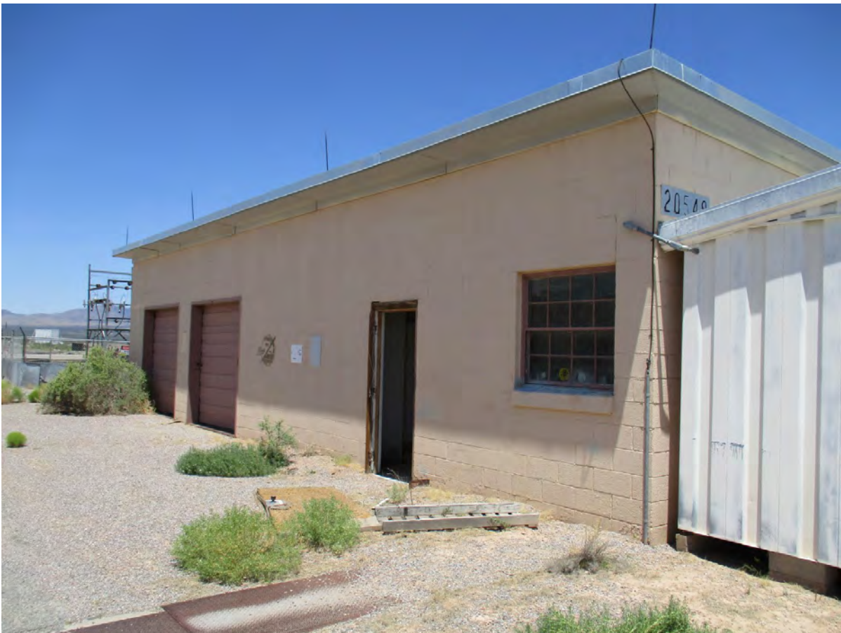
Figure 87. Property 20548 Generator Building, south and east elevations, view to the northwest.
