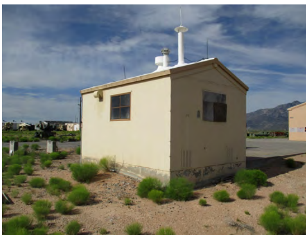
Figure 162. Property 21752, south and east elevations, view to the northwest.
