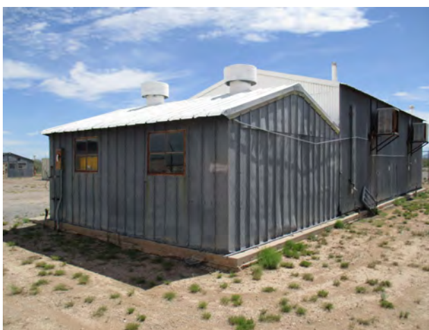
Figure 146. Property 21731, west and south elevations, view to the northwest.
