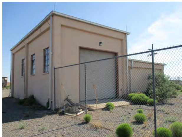
Figure 73. Property 20541, south and west elevations, view to the northeast.
