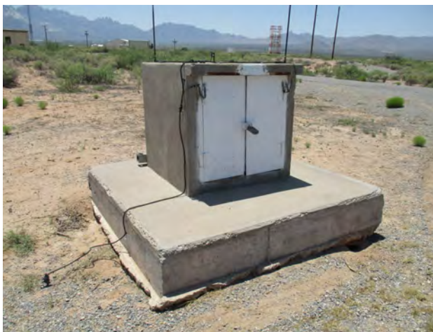
Figure 137. Property 34932, east and south elevations, view to the northwest.
