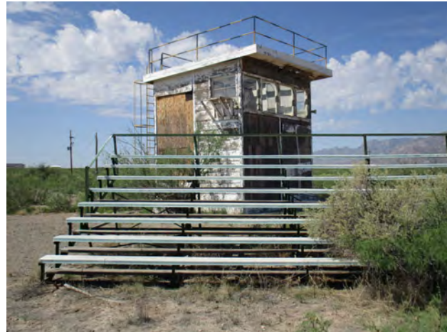
Figure 201. Property 20562 and associated bleachers, view to the southwest.
