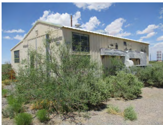
Figure 115. Property 20526, south and west elevations, view to the northwest.
