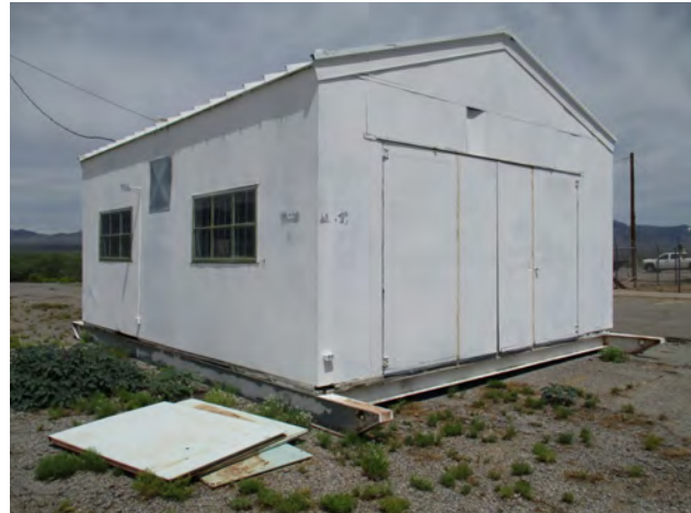
Figure 172. Unknown Portable Building 4, east and south elevations, view to the northwest.
