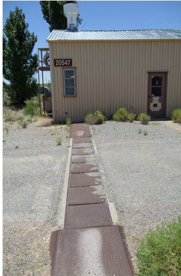
Figure 82. Cable trench that connects Properties 20547 and 20548, view to the south.
