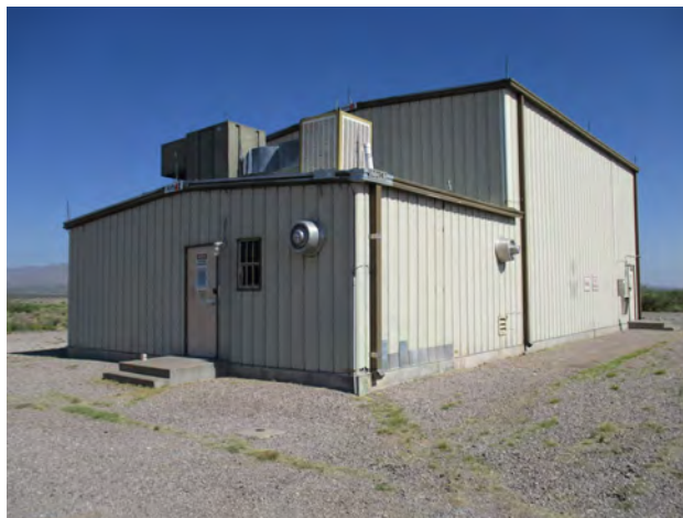
Figure 131. Property 20740, south and east elevations, view to the northwest.
