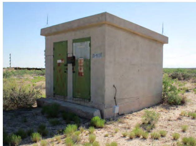
Figure 110. Property 20515, west and south elevations, view to the northeast.
