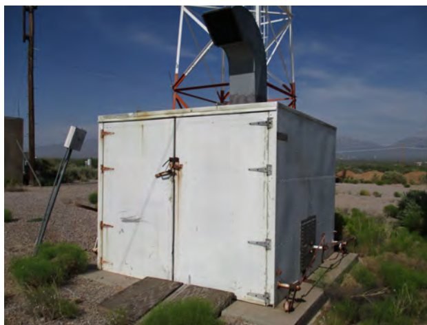
Figure 188. Property 25991, east and north elevations, view to the southwest.
