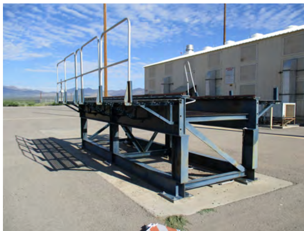
Figure 104. Hera Missile Assembly Stand, view to the northwest.
