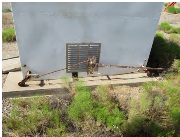
Figure 189. Property 25991, roller mechanism on north side, view to the south.
