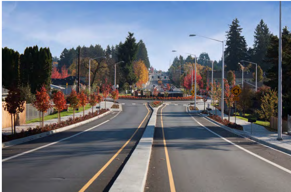
Vancouver: NE 137 th Avenue Roundabout
