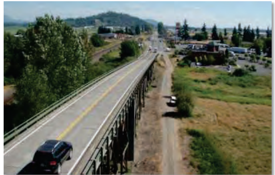
FIGURE 3: SKAGIT COUNTY'S BNSF BRIDGE REPLACEMENT PROJECT IS EXPECTED TO BE COMPLETED IN SPRING 2018. PHOTO CREDIT: SKAGIT COUNTY.
