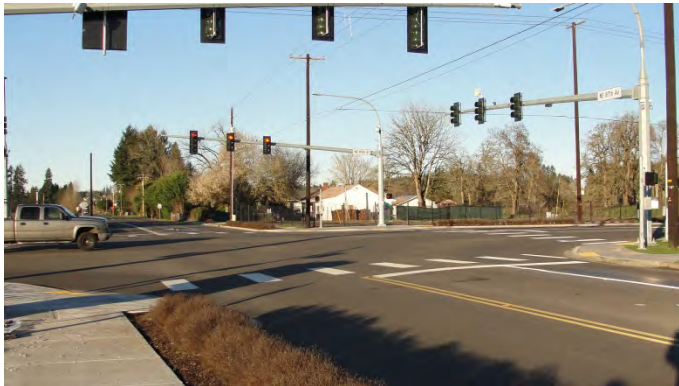
Clark County: NE 119 th Street/87 th Avenue Intersection
