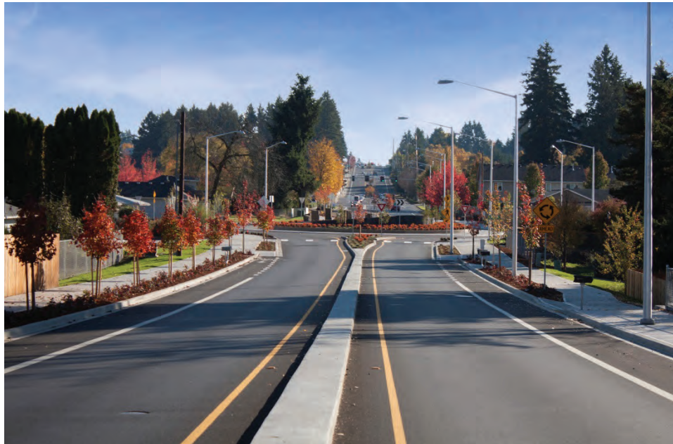
Vancouver: NE 137 th Avenue Roundabout
