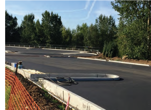
C-TRAN: Fisher's Landing Transit Center Expansion
