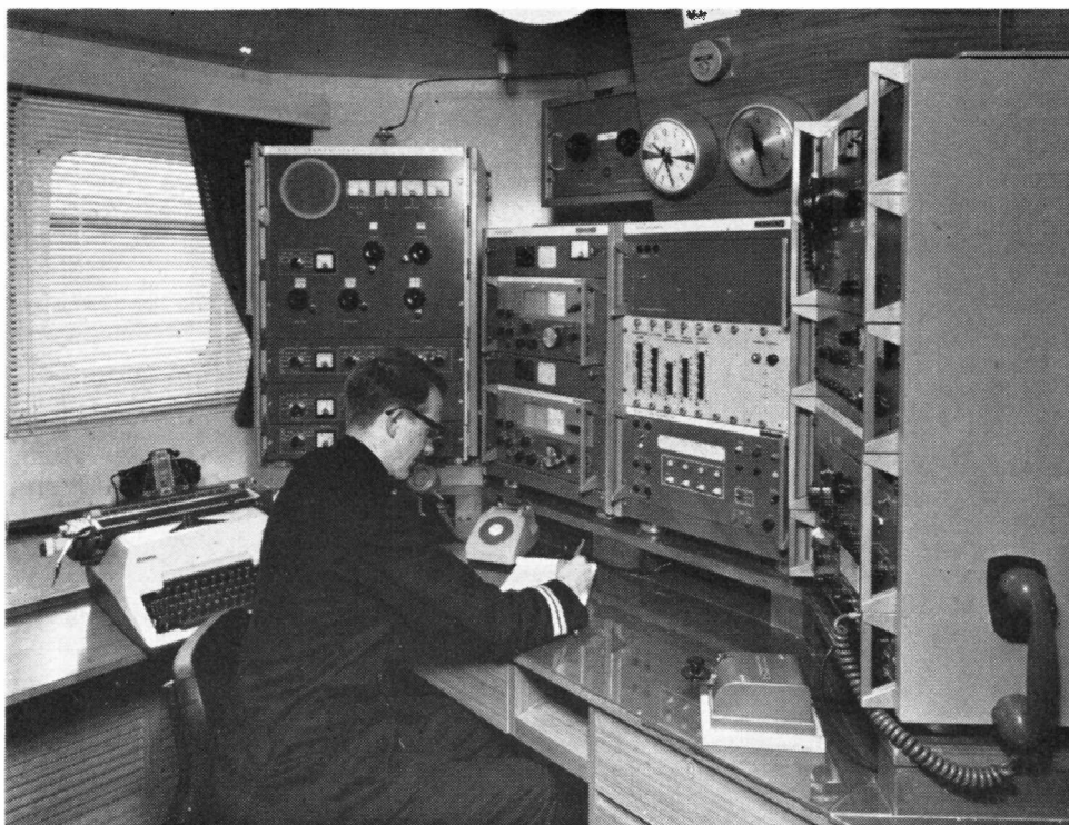
Radio room of the 24,000-ton container ship "Atlantic Causeway", signing GZML on the commercial frequencies. She is fitted with the most modern and sophisticated radio equipment supplied by the Marine Division of Redifon, Ltd. The main Tx can be set up on any of 195 channels in all marine bands, and it can put 1.2 kW into the ship's antennae on any of these frequencies. With the Redifon R.408 receiver this guarantees virtually world-wide communication. In charge of Redifon Marine training is A. F. Ward, G3HSP.
