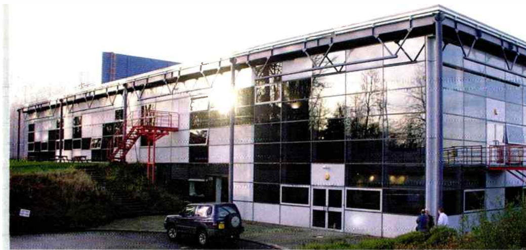
The ultimate Linn Product is arguably its Waterfoot factory. Designed by Richard Rogers, it's located on a 20-acre site on the south side of Glasgow
